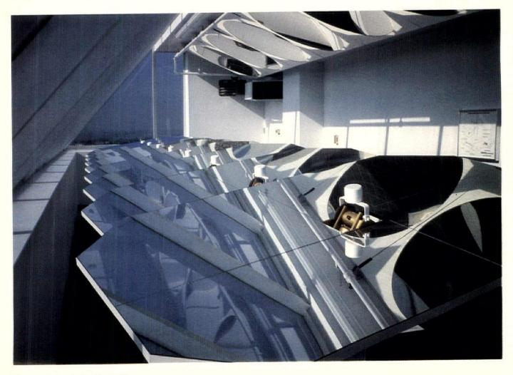
that, with a wider conduit, the light pipe could be used for as many as 10 floors of a building. The heliostats are essentially heavily silvered flat mirrors that measure 47 inches by 72 inches and are 2 millimeters thick. They are arranged in a straight line in a solarium, on fourfoot centers. A computer system calculates the position of the sun to ensure maximum capture of sunlight and controls the two-axis drive units.
