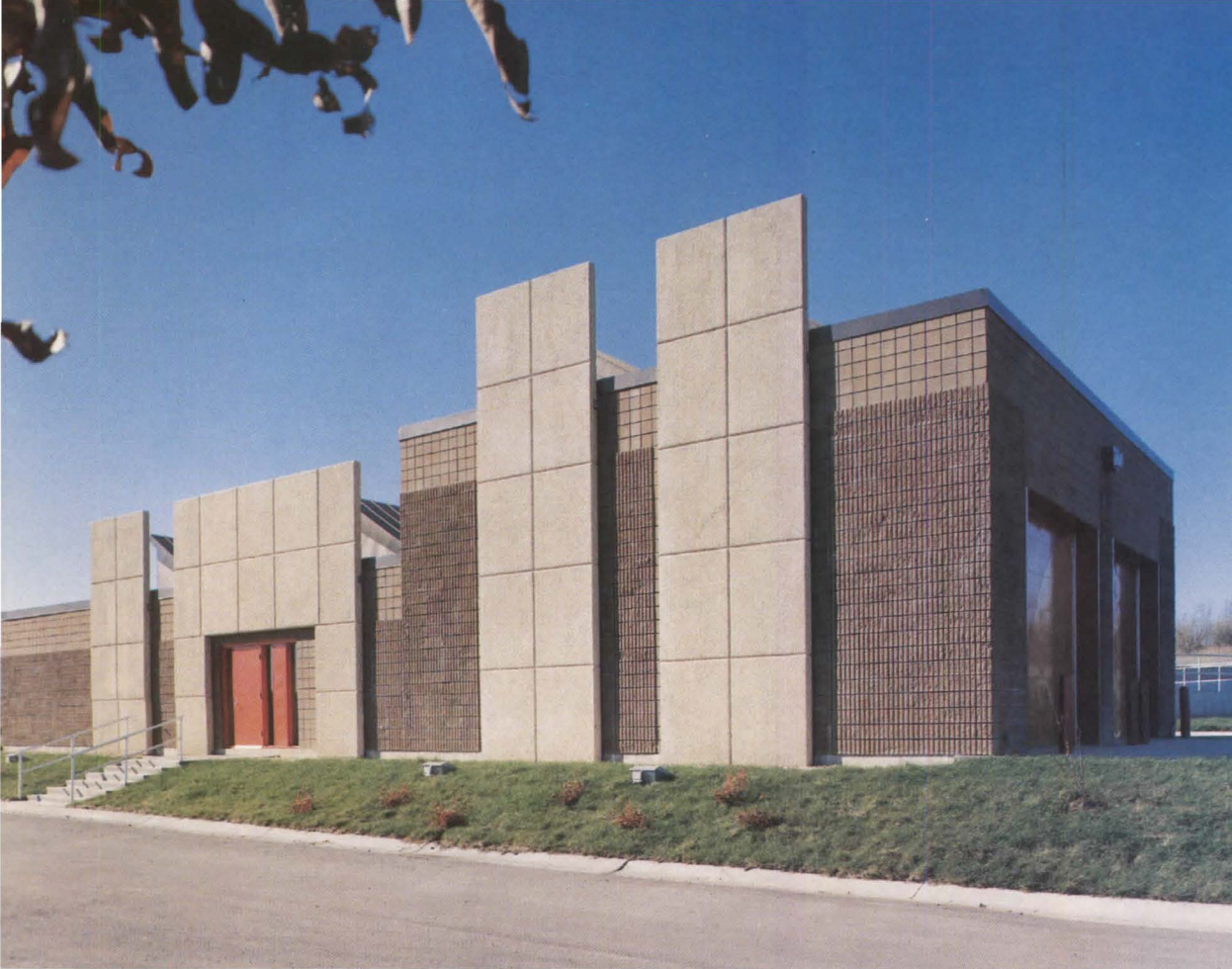
The complete building showing the split ribbed and scored concrete masonry units used for the exterior.
