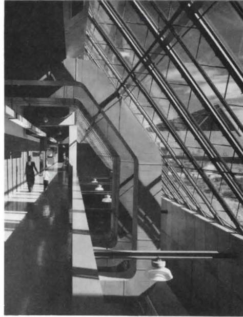
The North Campus of the Community College of Denver, by John D. Anderson Associates, uses 35,000 square feet of solar panels. From "Climate and Site." Architect's Handbook of Energy Practice.
