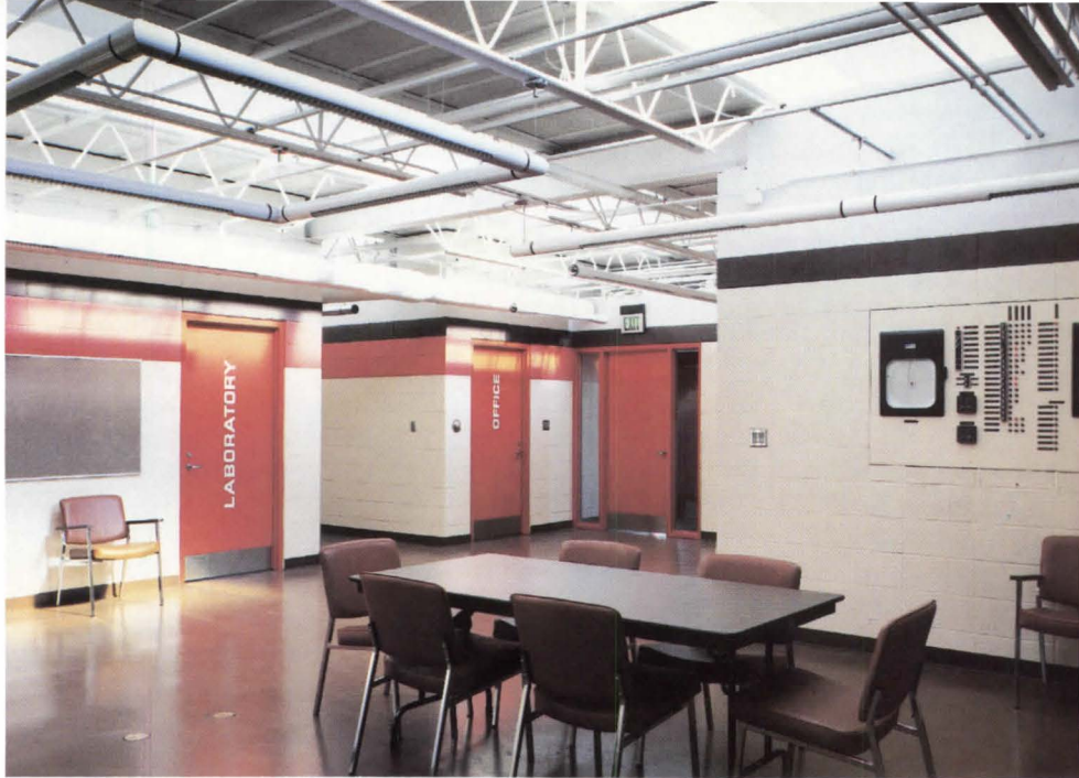
An interior scene with exposed concrete masonry walls used for heat storage and the clerestories above.
