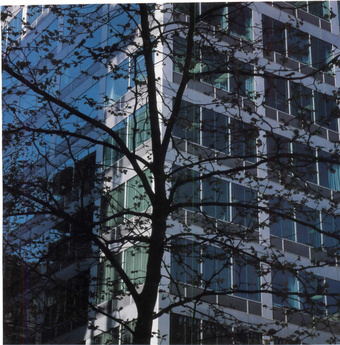
Left, the delicately detailed wall of the Equitable behind a delicate tracery of leaves and branches. Right, the building in its present context.
