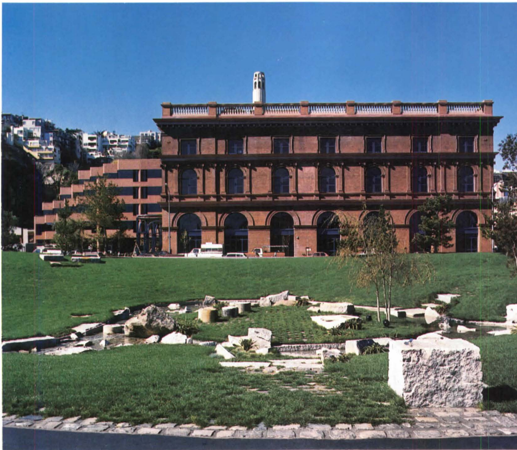
Right, the lower fountain and the beginning of the stream through the park. Grassy knoll (top) is sunk well below the level of surrounding streets. Above, the warehouse from the park.
