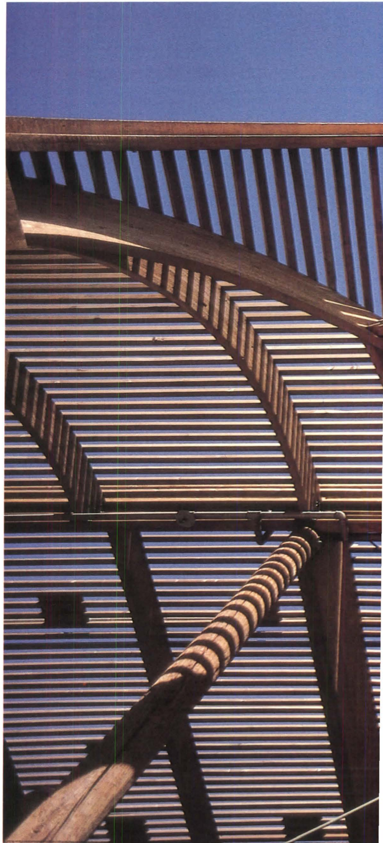
Wayne Thom Associates
