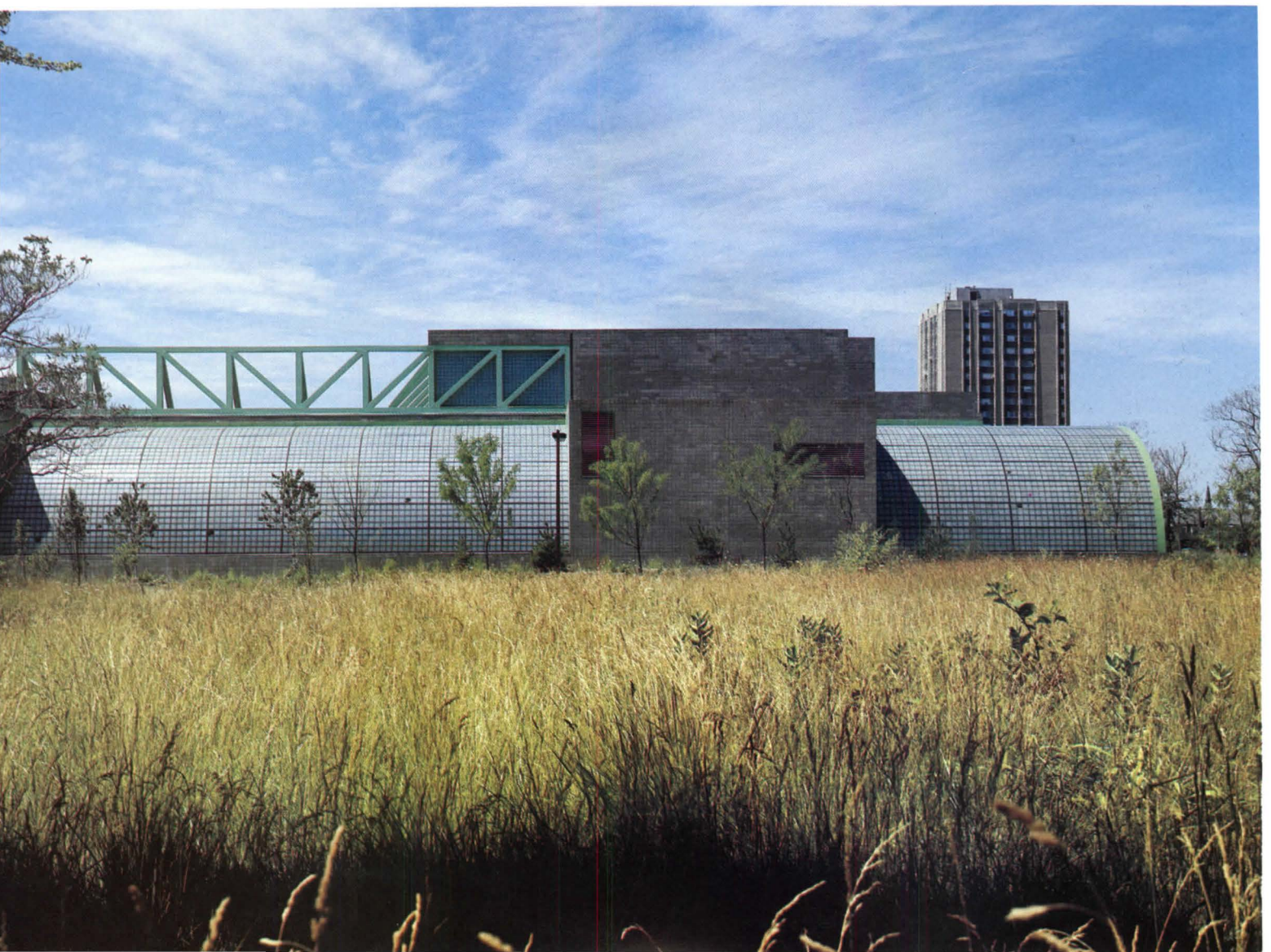
Irregular entrance facade, left, announces the modularity that is basic to the building design. A long facade away from the entrance, below, shows the vaulted boxing room at right and the half-vaulted swimming area, the latter spanned by an exposed steel truss above the roof.
