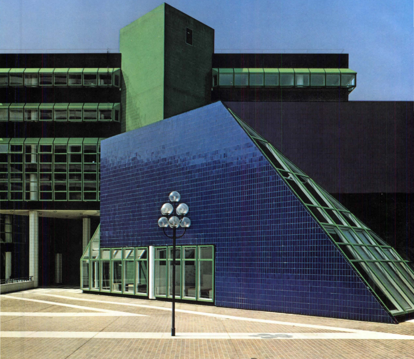
Cergy Pontoise Hotel, near Paris, clad in Monocolor #144 Intensive Blue and #143 Intensive Green. (Thin-set latex mortar on precast concrete.) Architects: Claude Vasconi and Georges Pencreach.
