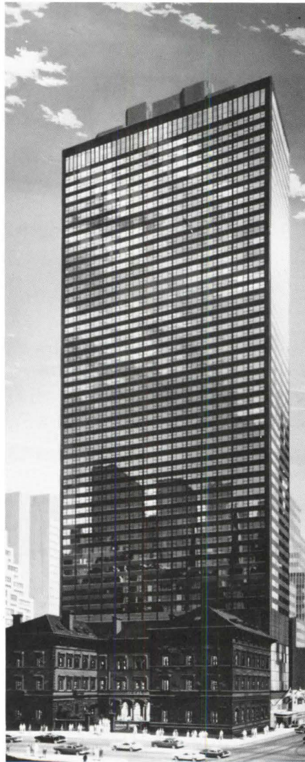
Architect: Emery Roth & Sons, P.C., New York Structural Engineer: The Office of Irwin G. Cantor, New York Contractor: Morse/Diesel, New York Owner: Helmsley-Spear, Inc., New York
