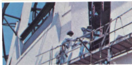
J-M panels were face mounted to steel dging, requiring about 25 per cent less ilation time than conventional masonry techniques.
