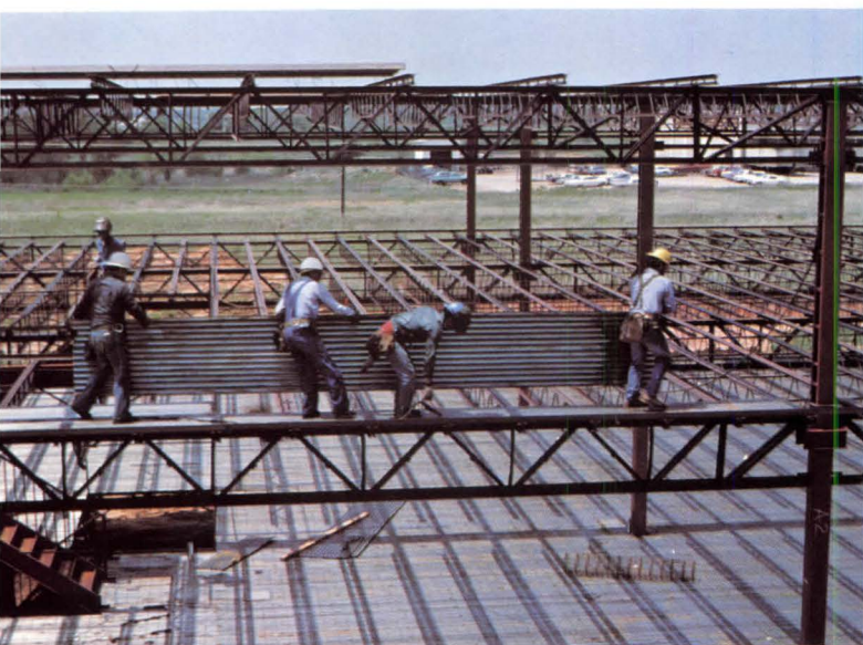
Vulcraft now manufactures a broad line of steel deck along with steel joists and joist girders.
