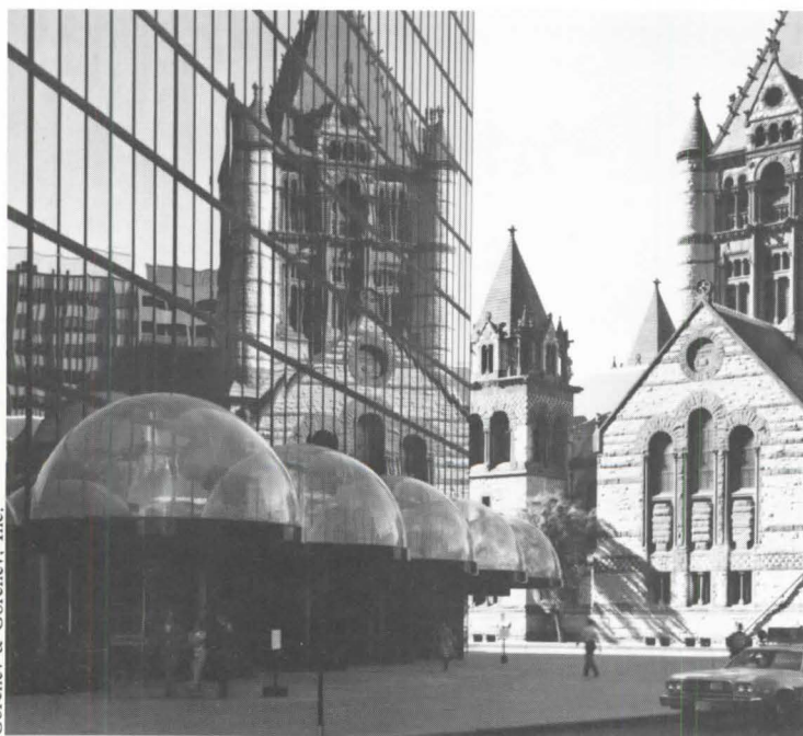
Canopies at the entrance, now removed, soon to be replaced.
