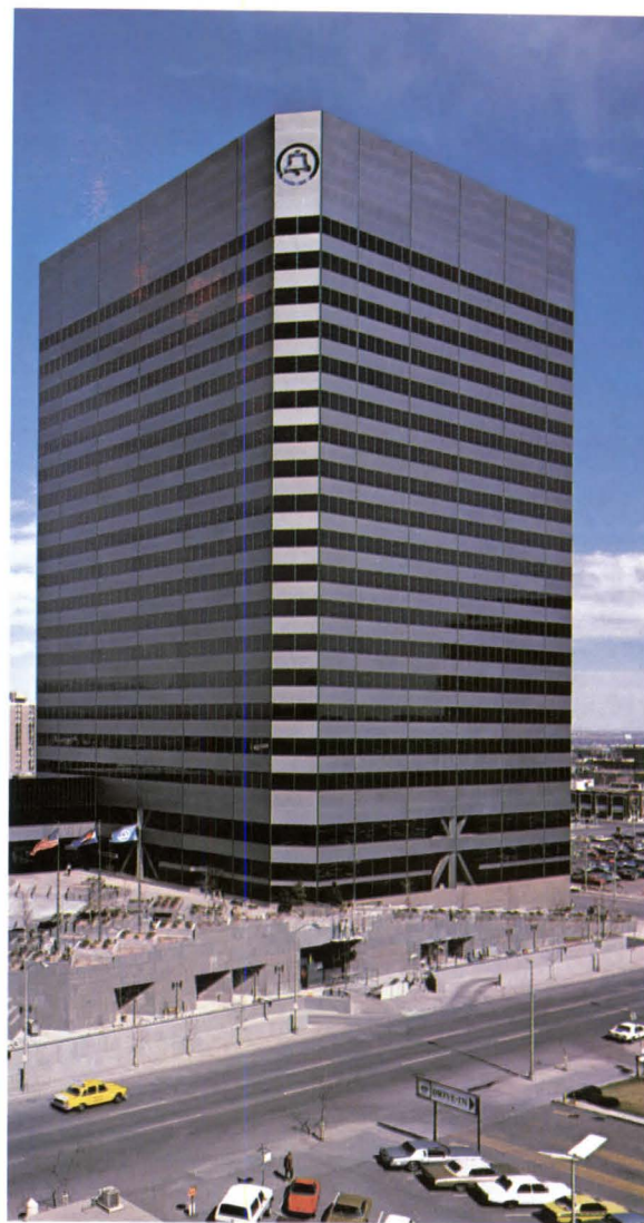
Aluminum sheet with Duranodic finish on the Denver Service Center of Mountain Bell, Denver, Colorado Architect: Rogers, Nagel and Langhart, Denver Metals, Division of Seagrave Corp., Minneapolis, MN Erector: PPG Industries
