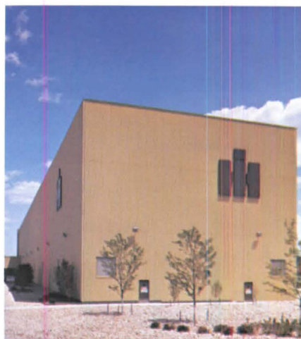
V-beam siding on the International Harvester Automated Materials Storage Facility at East Moline, Illinois Architect: Duchscherer-Obeist Associates Erector: Wisconsin Bridge & Iron
