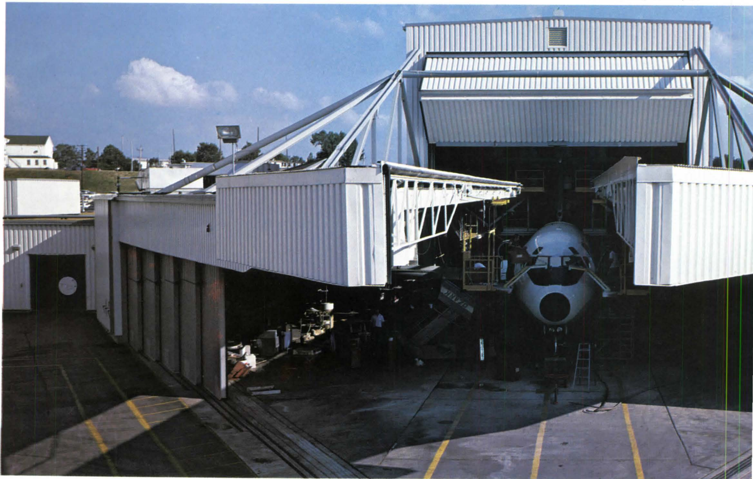
Bold Rib II siding at work on maintenance hangar for Ozark Airlines, St. Louis, Missouri Architect: R & D Contractors, Inc., Park Ridge, IL Erector: Stupp Brothers Bridge & Iron Company, St. Louis, MO
