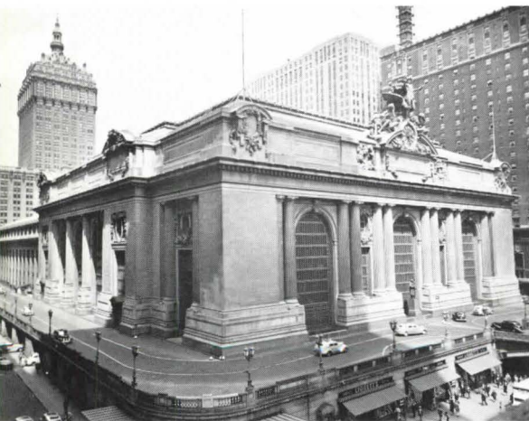
In a landmark decision, the U.S. Supreme Court ruled against building a tower over Grand Central Terminal (above). Union Station, Nashville, Tenn., to be restored for office space by GSA (right).
