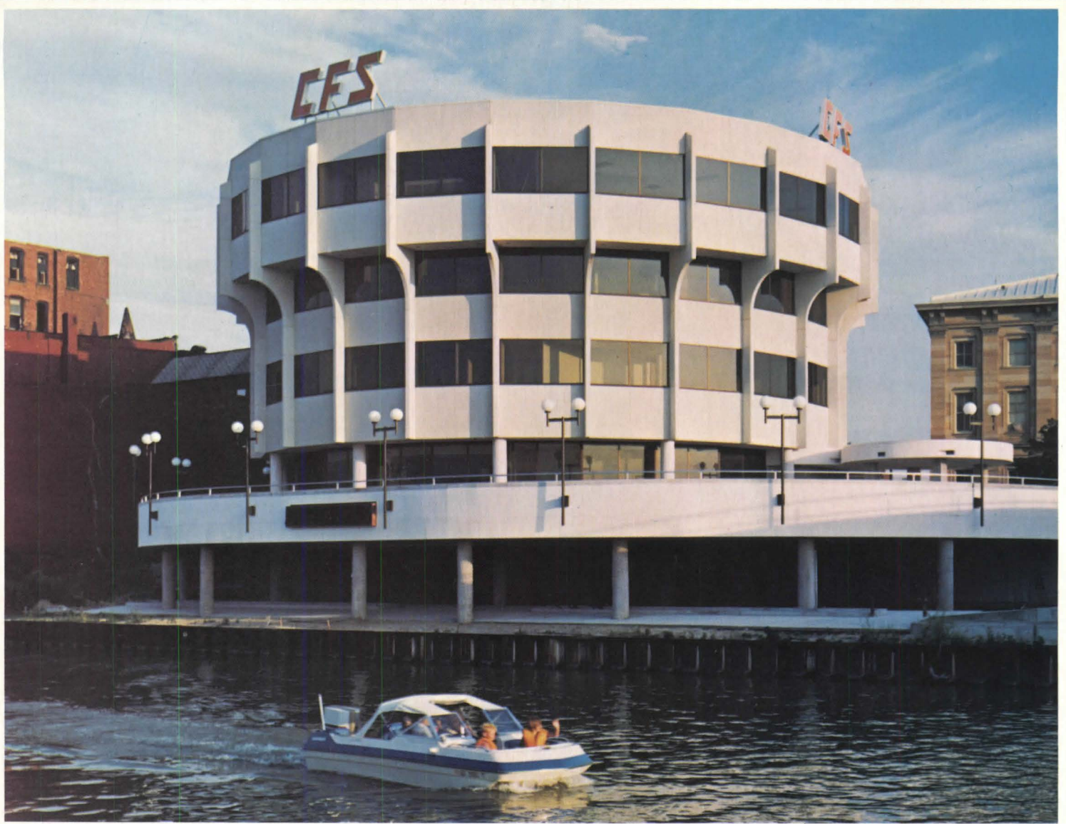
All supported floors are cantilevered to gain maximum floor area over the shallow site. The top floor has a diameter of 100 ft and overhangs the driveway below.
