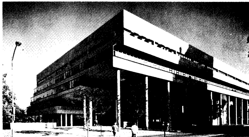
Gund Hall's famous greenhouse step section studio (top), surrounded on two sides by offices and classrooms (above). Opposite: the approach from the south.
