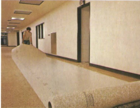
Rolls 6 feet wide and up to 90 feet long reduce seams to the minimum.
