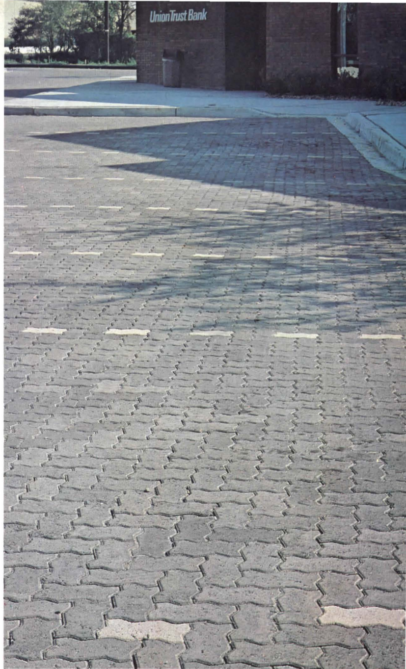
Parking area, Shopping Center, Baltimore, Maryland. Note that white units were installed to provide permanent parking space marking. Jewell Downing & Associates, Architects.
