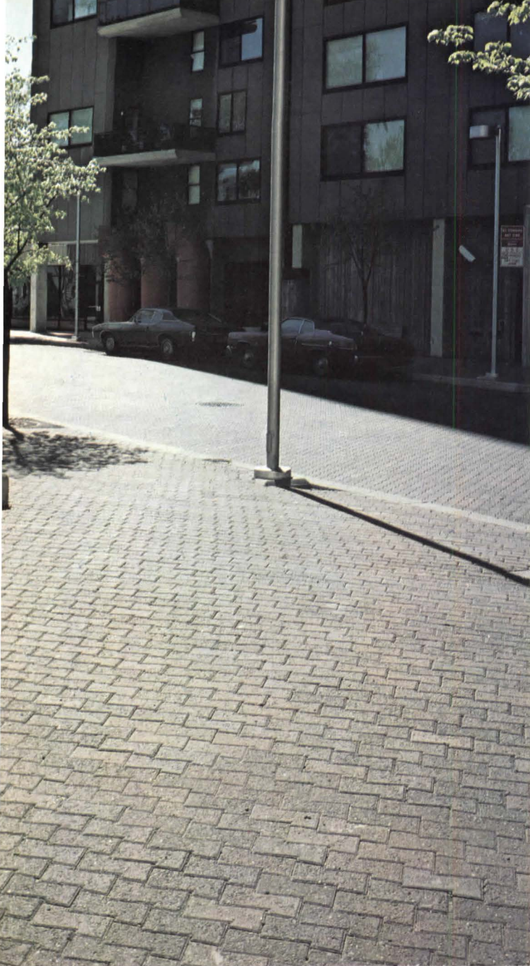
Roosevelt Island, New York City. This new town in the East River uses Concrete Pavers over a total area of 4\frac{1}{3} acres for both pedestrian and vehicular traffic. Installation has been in use since 1972. Zion & Breen Associates, Landscape Architect & Site Planners.
