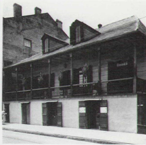
In warmer climates, living spaces were often on the second floor 'to catch the breezes,' as shown in Mme. John's Legacy, an early house in New Orleans.
