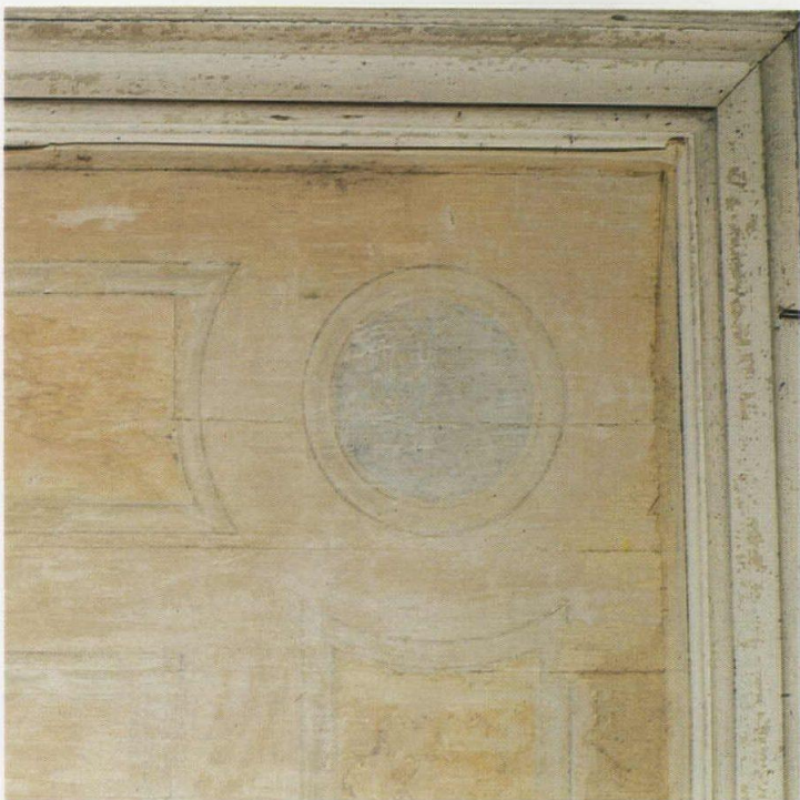
The dining room ceiling of the 1850s San Francisco Plantation in Reserve, La., required scraping away three layers of paint to find the original pattern (immediately above) before it could be restored by the author's firm to its glory (top).
