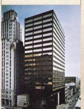
Bare USS COR-TEN Steel. When boldly exposed to the atmosphere, USS COR-TEN High-Strength, Low-Alloy Steel weathers to a dark, earthy color that only nature imparts. The oxide patina inhibits further atmospheric corrosion. Unlike most materials, its appearance improves with age.
