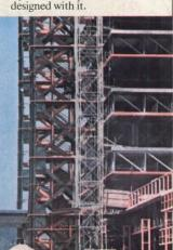
Flame-Shielding. Another fireprotection concept developed by U.S. Steel. Flame shielding eliminates having to cover perimeter structural steel members with fireproofing materials. Spandrels are protected by shields attached to the flanges of girders. The shields deflect the flames outward and away from the steel.
