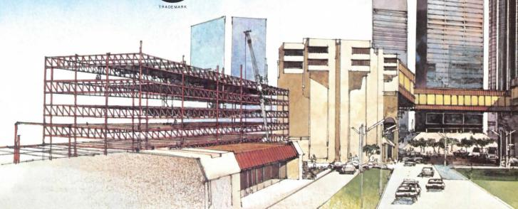
Interstitial Space Design. A series of structural steel sandwiches or full height service levels between working floors—in which mechanical, electrical communication lines and distribution and collection systems can be housed and maintained. Over the past 6 years, 35 hospitals have been
