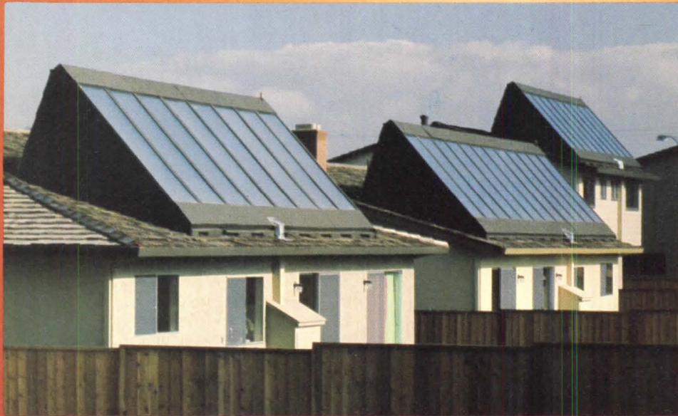
Solar heating development at Laurel Park East, Santa Clara, California, utilizing tempered Sunadex™ glass. Collector manufactured by American Solar King, Inc.
