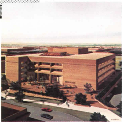
Federal Office Building, Topeka, Kansas. Uses mass plus heavy insulation in walls and roof to create an energy-conserving envelope. Open, skylighted interior atrium allows minimum exterior glazing. Windows comprise only 17% of exterior wall area. Glazing is recessed or shaded to reduce heat gain in summer. Lighting is 2.3 watts/sq. ft. Estimated saving on heating costs: $2,600/year.
