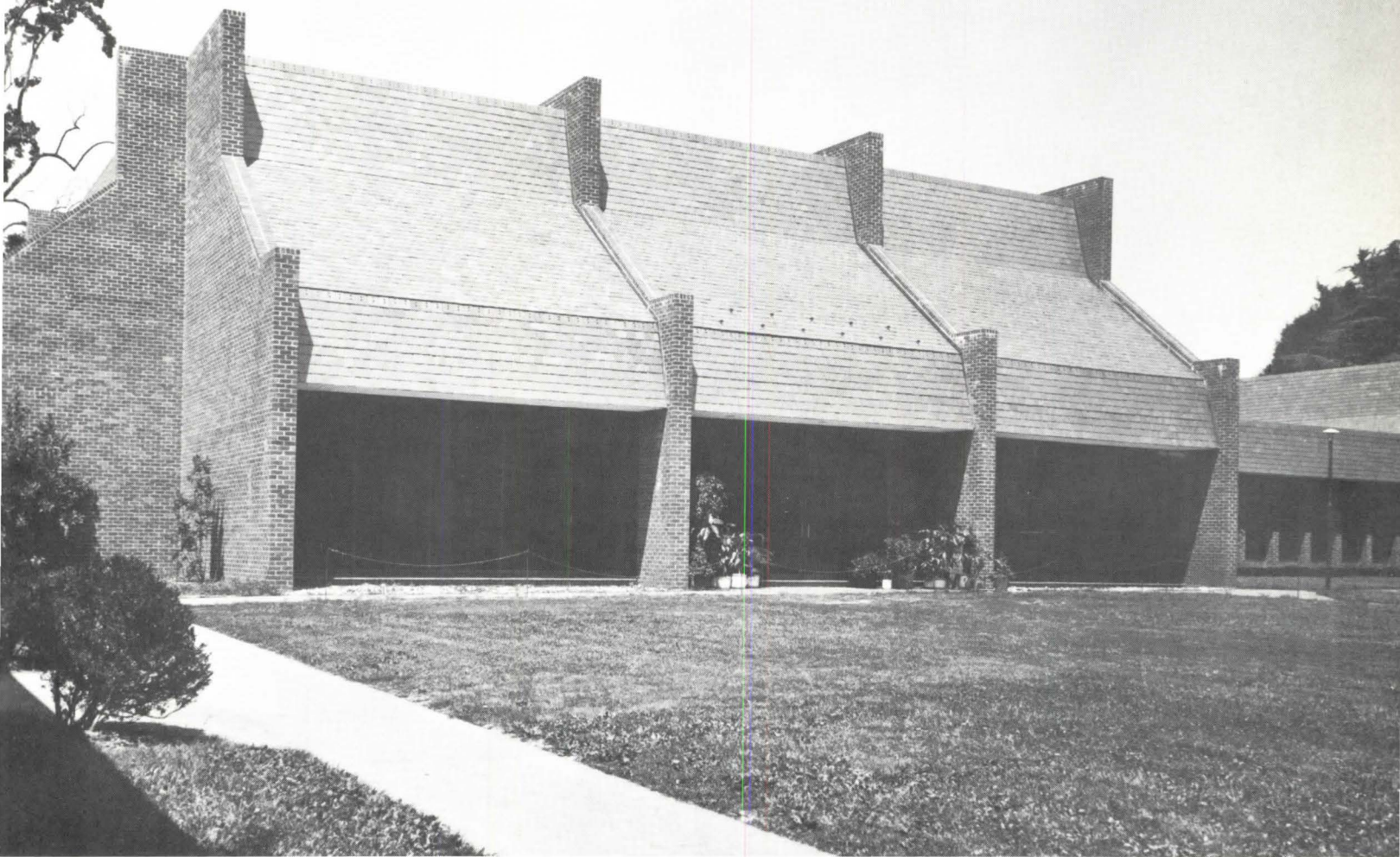
Library/Chapel building, St. Catherine's School, Richmond, Virginia • Architects: Hardwicke Associates, Inc., Richmond, Virginia Roofing Contractor: N. W. Martin Bros., Richmond, Virginia
