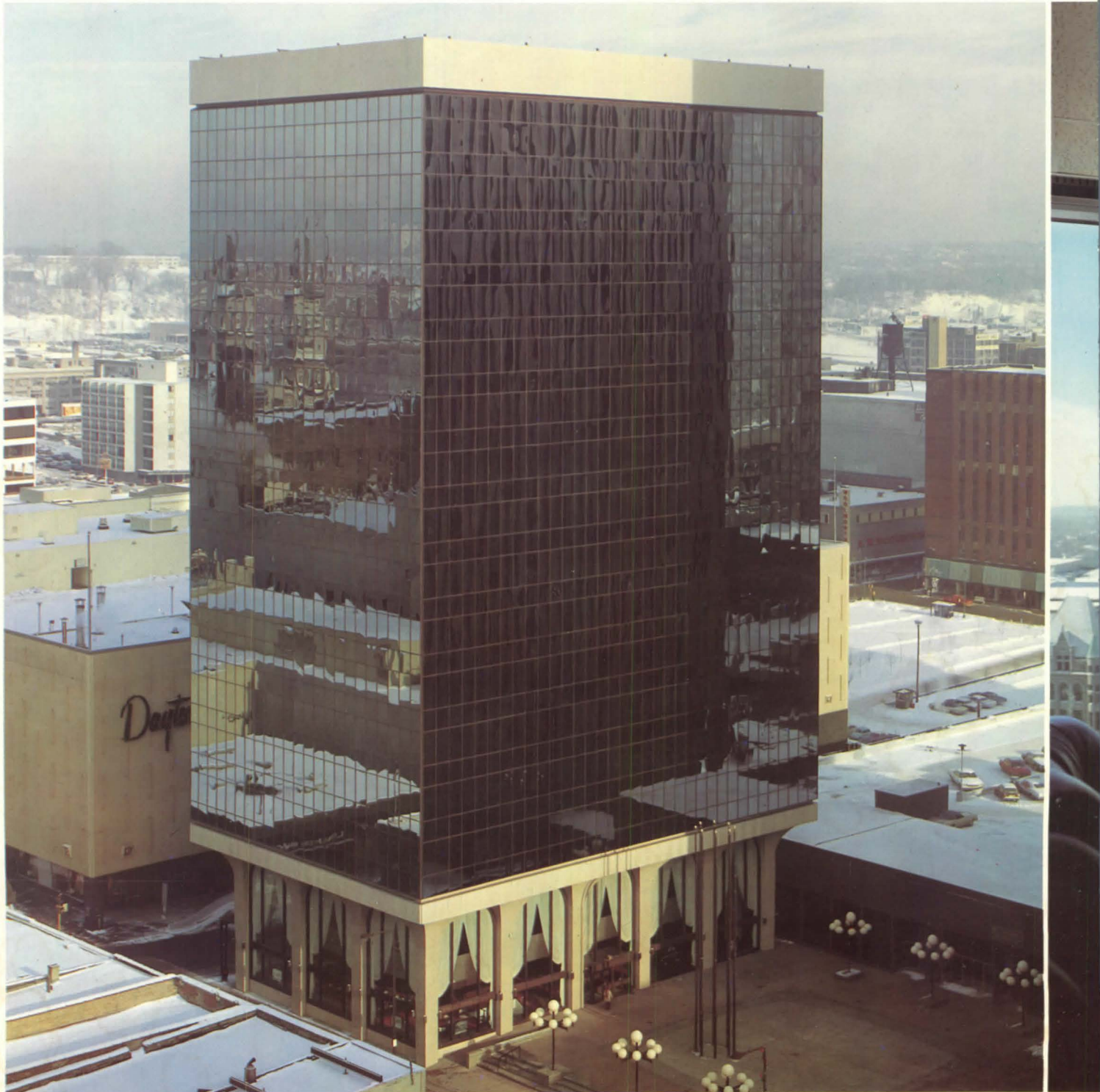
Northern Federal Building, St. Paul, Minnesota. Owner: Yorktown Investment
