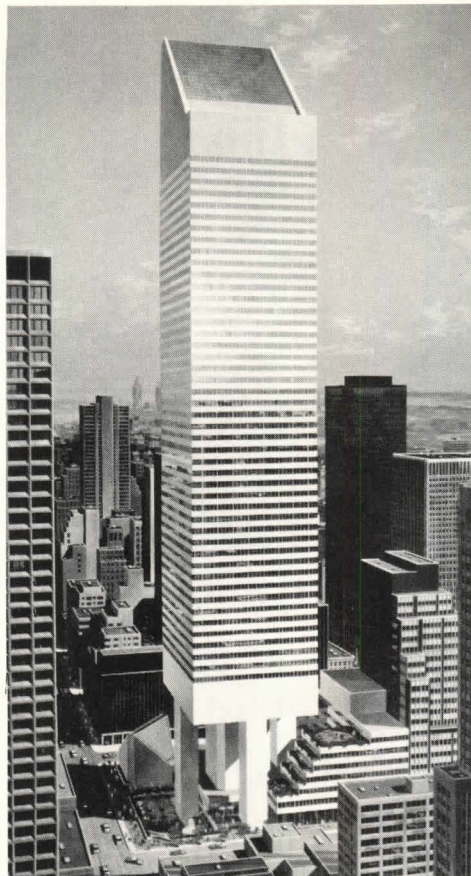
Shown here is a solar energy collector on top of the 56-story Citicorp Center, now under construction in New York City (Hugh Stubbins & Associates, Inc., with Emery Roth & Sons). If a Massachusetts Institute of Technology research team finds the design feasible, a flat-plate collector mounted on the south-facing sloping roof would operate a dehumidifier in an airconditioning unit.
