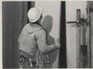
2. Installing core panel.
