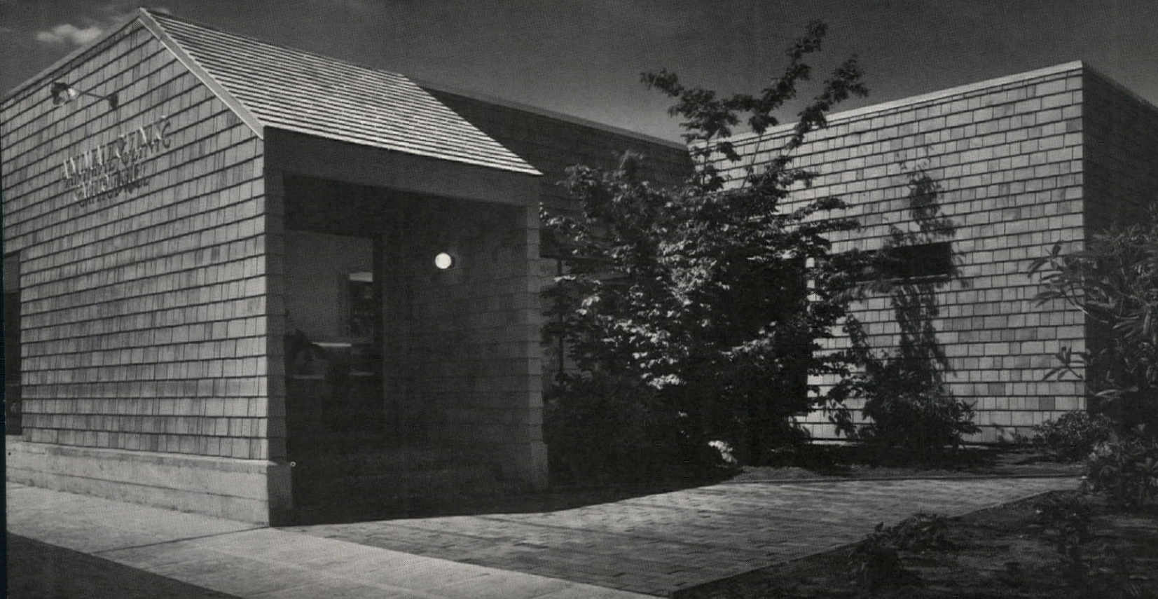
Animal Clinic, Seattle, Washington Certigrade Shingles No. 1 Grade, 18" Perfections. Architect: Robert Mesher, Gerald H. Kumata & Partner
