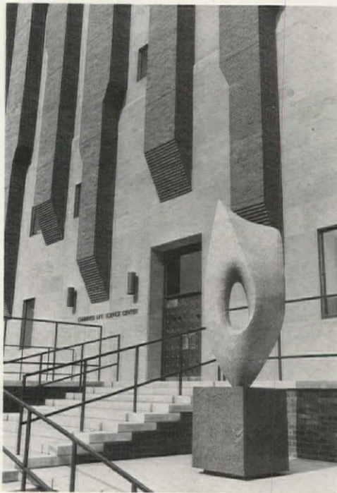
Forty chimneys serve as exhaust towers on the University of Chicago's Life Science Center. Sculpture adorning the front entrance is by Antoine Poncet.
