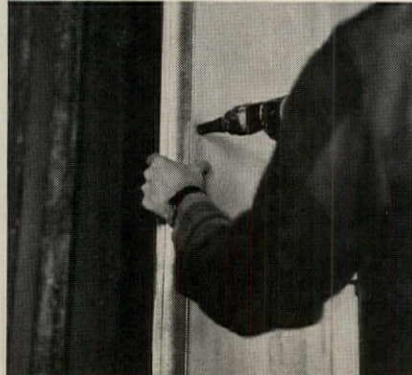
3. Attaching core to T-spline.
