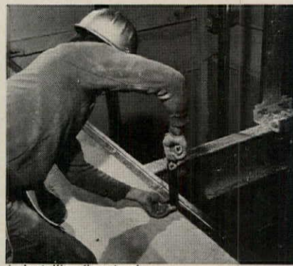
1. Installing floor track.
