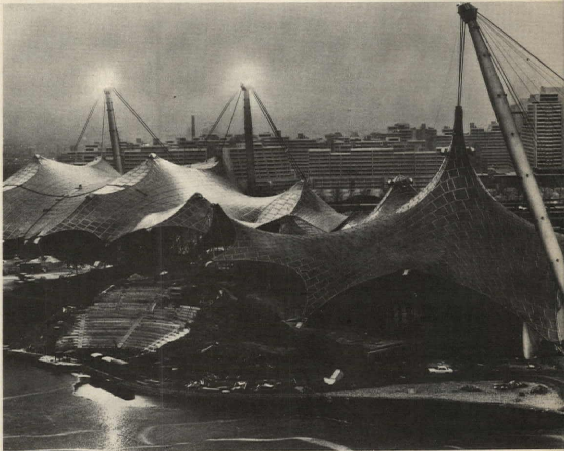
The gymnasium and swimming pool are covered by a tent; an artificial lake and a stage are in the foreground (above). Olympic Village (below left) houses competitors and other personnel.
