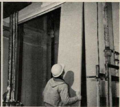
2. Installing core panel.
