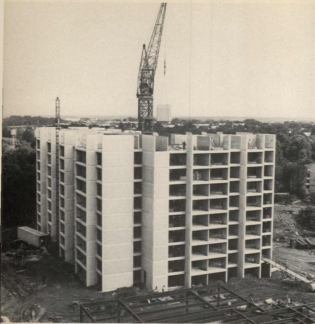
An exterior wall panel goes up and, finally, the white sand and concrete University of Delaware Student Living Center is topped out.
