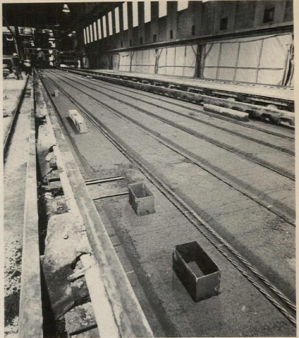
Styrofoam insulation is positioned on top of concrete in a wall panel (a third layer is reinforced concrete and serves as the components' structural element). Workers pour finish layer of concrete in a wall form. Tension cables and penetration forms are positioned in floor slabs.
