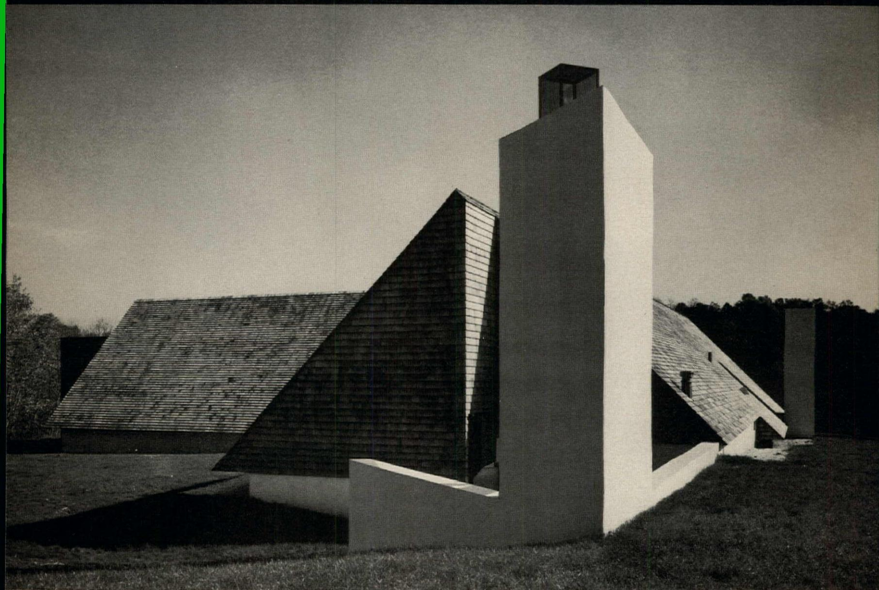
Girl Scout dining hall, Quakertown, Pennsylvania. Certigrade shingles No. 1 Grade, 18" Perfections. Architect: Frank Schlesinger FAIA.
