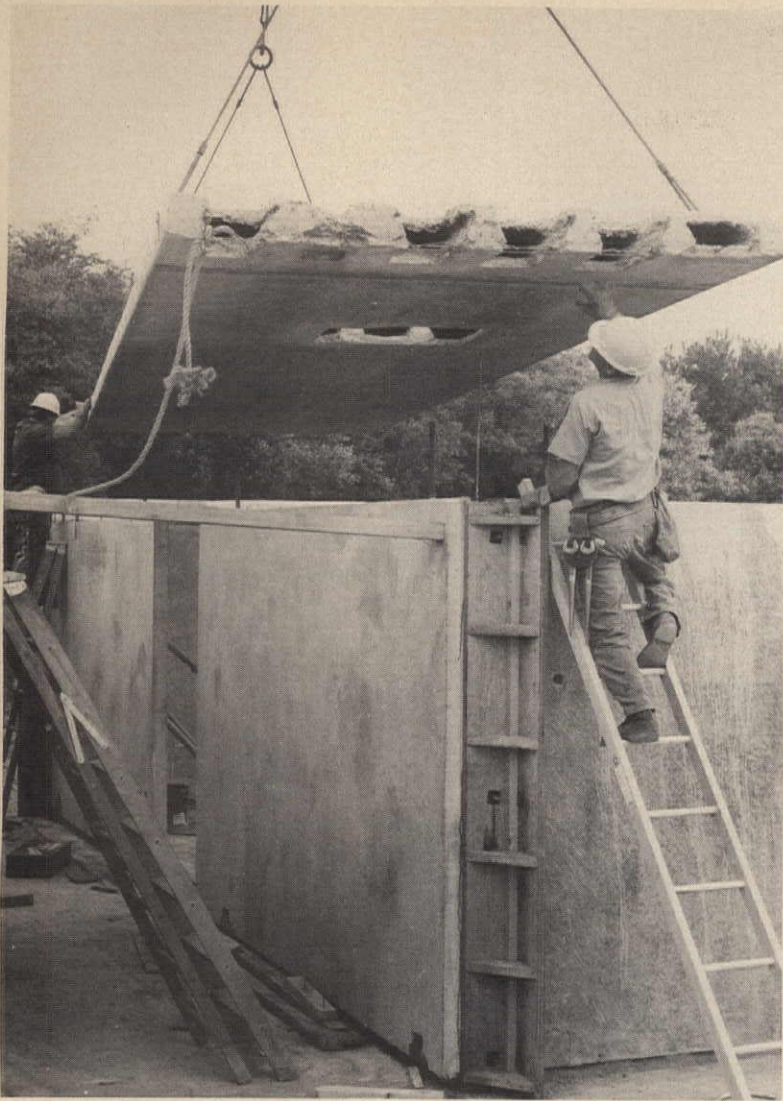
Hollow-core floor/ceiling unit is guided into place; loops of reinforcing steel bar exposed at its end will be placed over steel dowels cast in walls; the wooden forms are used while concrete in the joints is drying. A precast one-story high stair unit is being installed.
