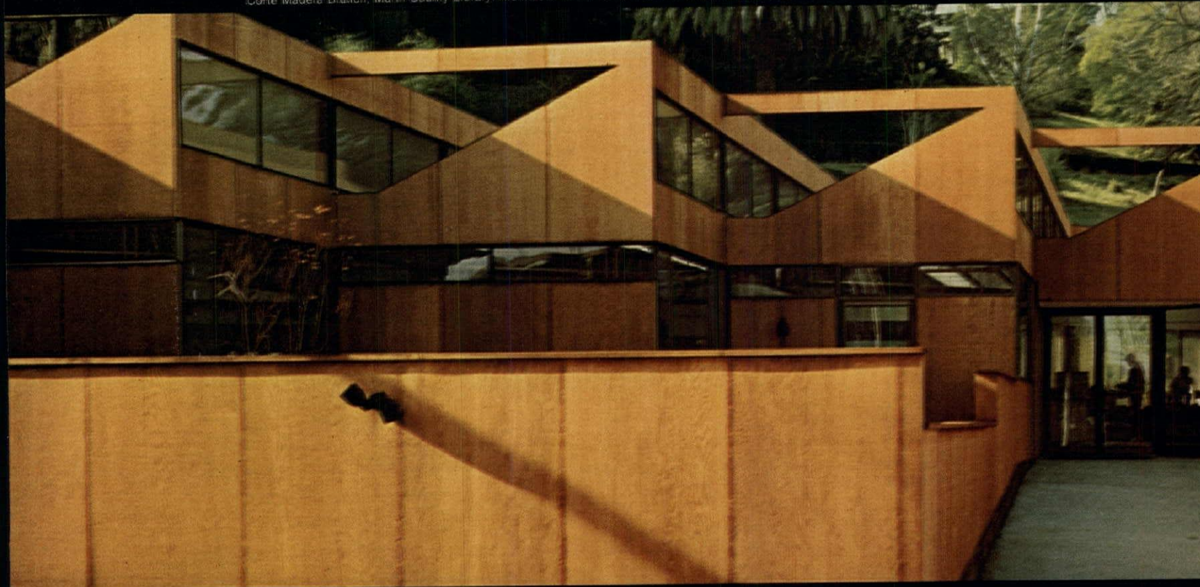
Corte Madera Branch, Marin County Library. Architects: Smith Barker Hanssen, A.J.A., San Francisco, Calif.
