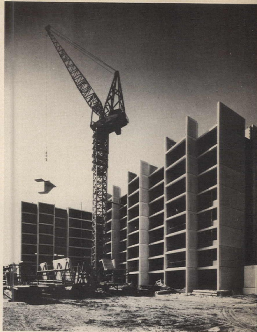
Hollow-core floor/ceiling unit is guided into place; loops of reinforcing steel bar exposed at its end will be placed over steel dowels cast in walls; the wooden forms are used while concrete in the joints is drying. A precast one-story high stair unit is being installed.
