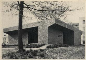
Gainesville Area Chamber of Commerce, which uses precast brick soffits backed with reinforced concrete slabs for the 5-foot overhangs, contributes to the improvement of the town.
