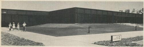
All access to manufacturing area can be controlled through one entrance. Glass-walled office facility is square in plan with an enclosed courtyard in the center.
