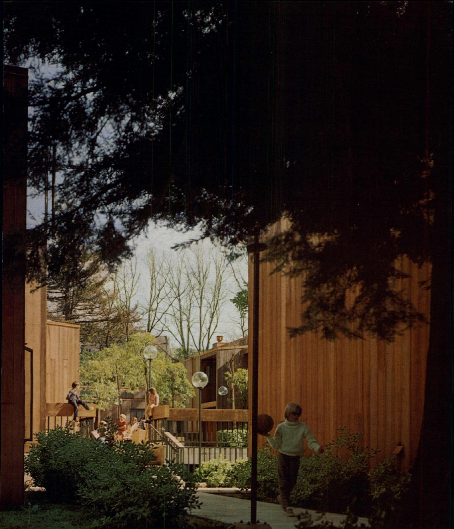
Married student housing, Theological Seminary, San Anselmo, California Architects: Frants Albert, AIA and Wm. M. Abend, AIA, San Francisco.
