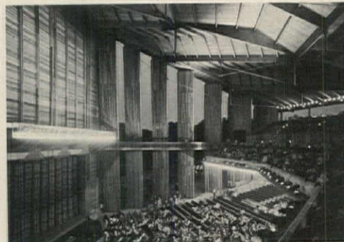
Unfinished wood roof of Center, springing out of hillside, covers 23,000 square feet.
