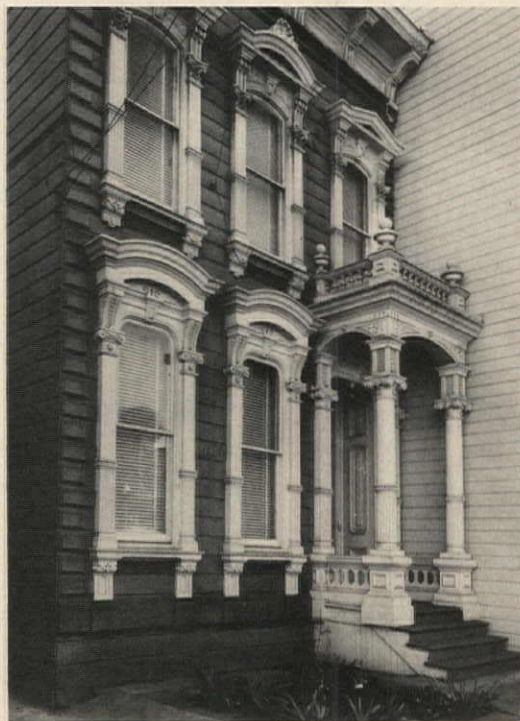
Facade, Western Addition
