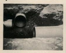
P.V.S. duct is trucked to the job site like this . and stored in the open as seen at right. It is un-affected by water, cold, heat or atmospheric fumes.
