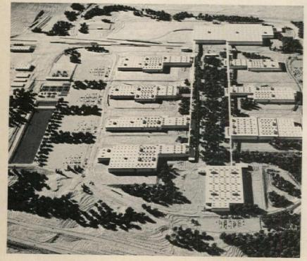
General Electric Company Appliance Park-East, Columbia, Maryland, is under construction on an 1,100-acre site. The movement of raw material is from the peripheral end of the manufacturing buildings to the opposite end facing the central mall, from where the products are carried by overhead conveyor to the warehouse for shipment and storage. Office buildings are underneath the conveyor enclosure, allowing them, as well as employee cafeterias, to overlook the parklike mall.
