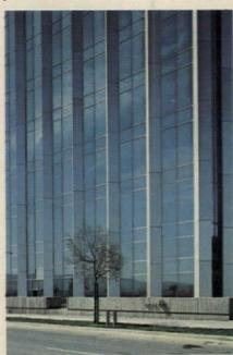
The improved 'U' value of the double glazed glass had a significant effect on reducing the size — and cost — of the heat recovery cycle required by all-electric concept.
