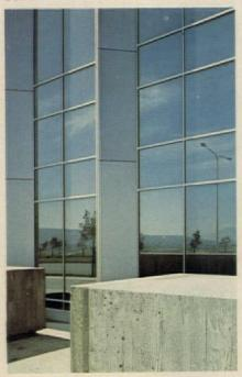
The reflective glass increased rentable area on the upper 15 stories due to smaller fan-coil machinery on each floor. The estimated rental area gained was 3% of total on these floors, representing rental income of \$46,656 per year. The additional rental income, and owning and operating cost savings, total \$66,478 per year. If this amount were capitalized at 10%, an initial investment of \$664,780 could be justified.
