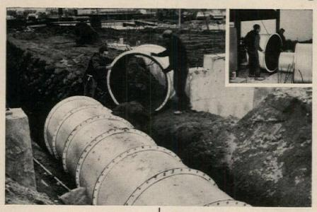
P.V.S. 42" spiral rolled duct meets at plenum head. The P.V.S. coating prevents corrosion from ground water, and is impervious to acid or salt attack from mineral elements in the soil
