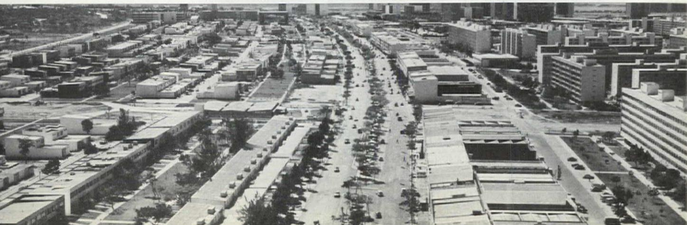
Main business street has private duplexes on one side (left), stores on the other. All homes face front to front.
