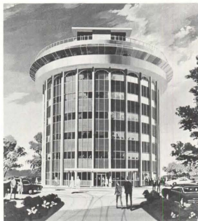
Good place for a drink: building encloses a million-gallon standpipe.
