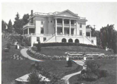
Typical of the grander Colonial Revival houses of the first part of the century is the Josselyn House.
