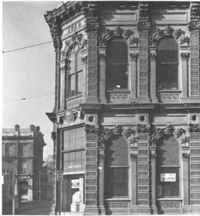
Ironwork from Ladd & Tilton Bank, 1868, is incorporated in Ladd & Bush Branch of United States National Bank, Salem, Oregon. It was perhaps the finest of cast iron facades.
