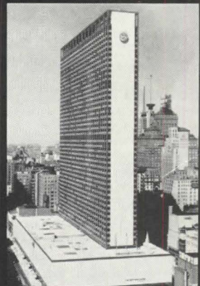
NEW YORK HILTON William B. Tabler, Architect
