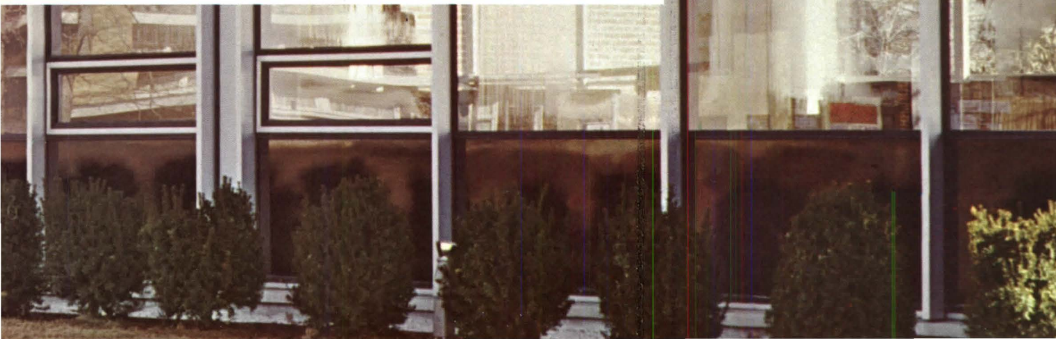
Zipperwall 2: double Neoprene design for 1/4" plate glass.
