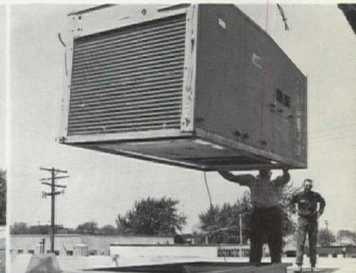
All-weather unit bolts to frame, needs no other sealing.
