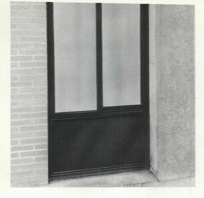
Window wall for an apartment or commercial building. Fluropon adds the dimension of long-lasting color to exterior designs. Roll coated or sprayed onto metal, Fluropon won't chip, shatter or delaminate.
