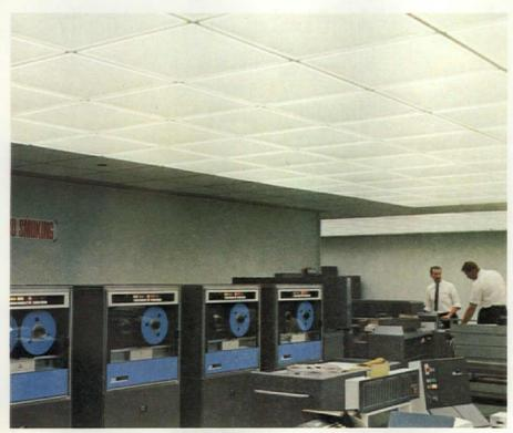
Where visual accuracy is essential, polarized lighting plays a key role. The Pennsylvania Railroad Company installed a POLRIZED lighting system in the computer area at its midwest ticket reservations facility in Chicago. The uniform low-brightness and reduced glare produce a high degree of visual comfort and efficiency. A similar installation of standard (non-polarized) lighting would have to be increased to approximately double the foot-candles to equal the visual effectiveness achieved here.
