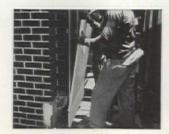
Horizontal supports lock into grooves in edge of 7/8" marble.
