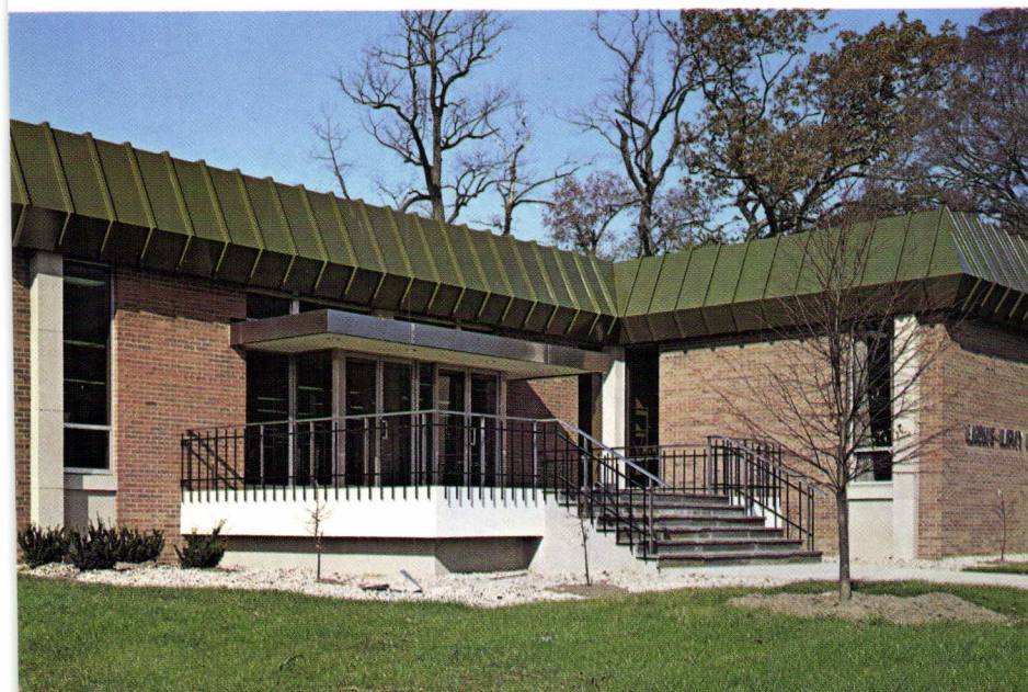
Porcelain enamel panels serve as both fascia and coping on campus library.
