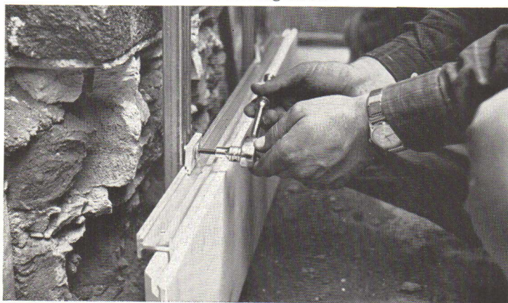
Horizontal members fastened by special clamps.
