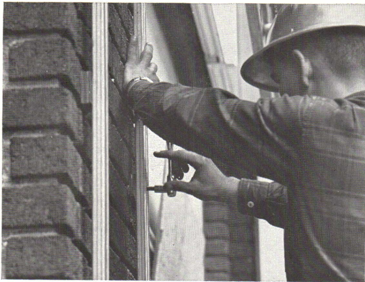
Vertical struts are anchored to existing facade.
