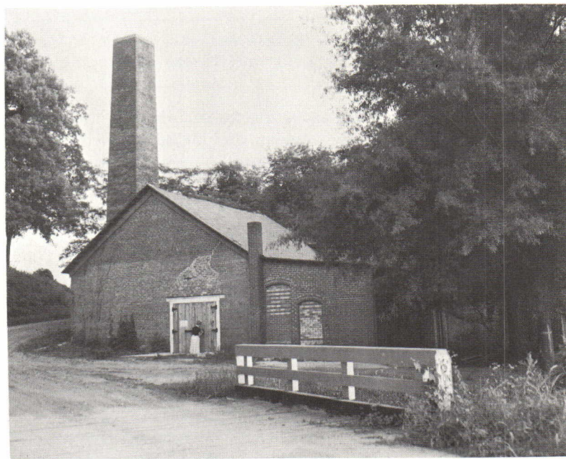
Another North Carolina pumping station becomes an Arts and Science Museum, with a storeroom theater.
