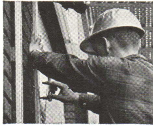
Vertical struts are anchored to existing facade.
