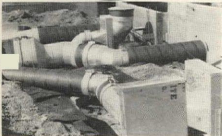
SONOAIRDUCT Fibre Duct fits all standard aluminum or galvanized steel bends, elbows, tees and registers.
