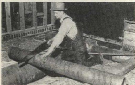
SONOAIRDUCT Fibre Duct can be cut to exact length on the job. Will not chip, crack, or break if dropped. More economical because every piece is usable.
