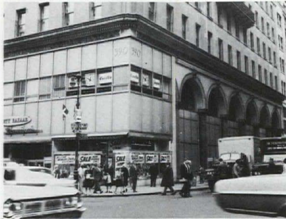
Fig 10a—Gorham building: “divided up the property for small stores and offices (10b) . . . a mutilation”
