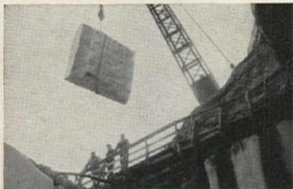
Outsize blocks of marble were taken from our Danby quarry for this installation. 250 slabs with random, non-matched veining were specified by architects Skidmore, Owings & Merrill.
