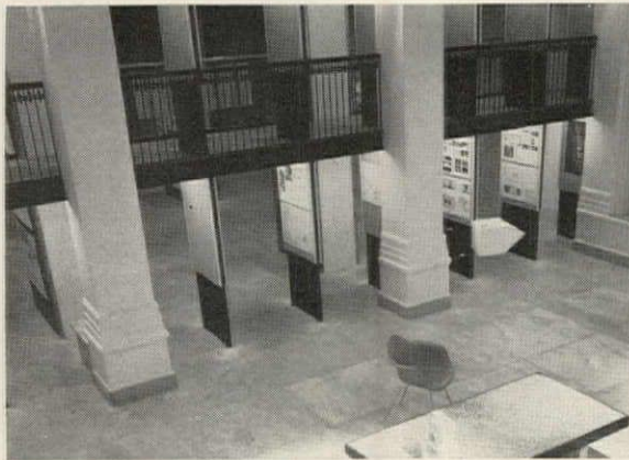
Main Exhibition Area: Columns from stacks that had to be retained for support have been used to create display areas in the lobby. They are surfaced with precast panels of different types of aggregate.
