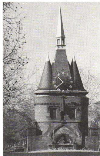
Gateway to Washington Terrace, one of numerous West End private developments—designed by George R. Mann
