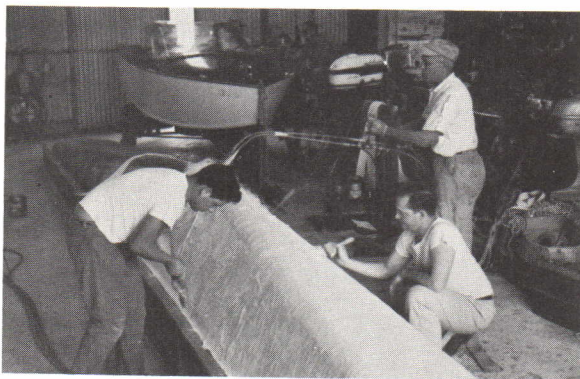
Spraying first full-size test unit
