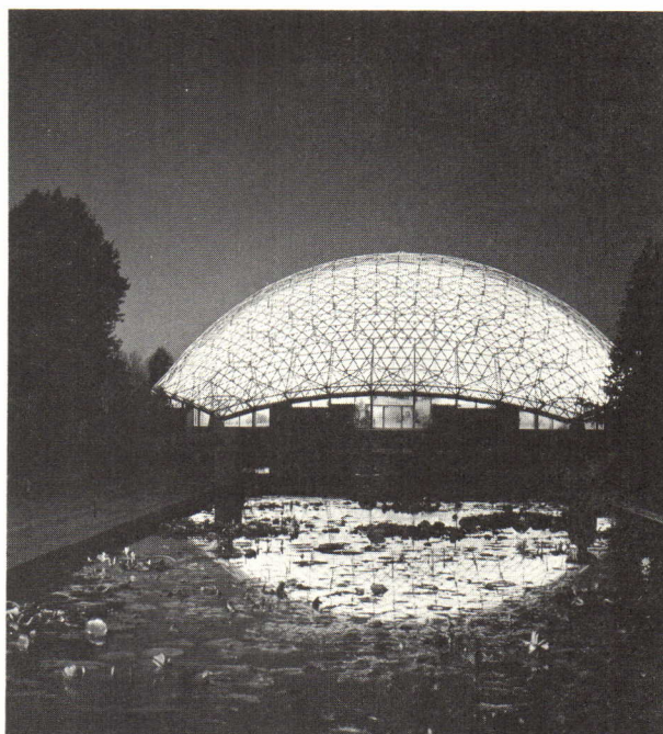
The Climatron, in the Missouri Botanical Gardens, is the world's first greenhouse to be completely airconditioned, with controlled temperature and humidity variations within an unpartitioned space 70 feet high and 175 feet in diameter
