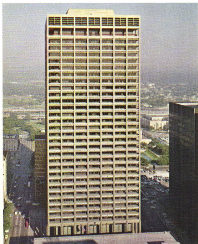
Tennessee Building: Houston, Texas. Architect-Engineer: Skidmore, Owings and Merrill, San Francisco, Calif. General Contractor: W. S. Bellows Construction Corp., Houston. Custom Curtain Wall Supplier-Erector and Kalcolor Applicator: Kawneer. Over 2,000,000 pounds of rich amber grey Kawneer aluminum hard color went into this job.
