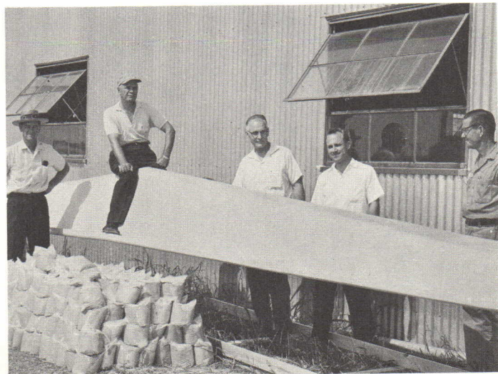
First unit ready for load testing
