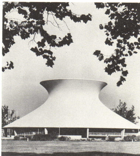
The St Louis Planetarium, a hyperbolic silhouette defined by a vertical axis around which straight lines revolve at constant angles to the axis. The flared upper section shields the observation deck from the city's lights
