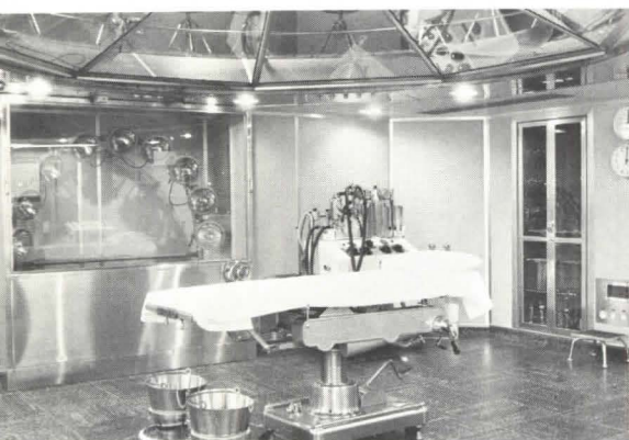
Operating theater, State University Hospital, Ghent. Flexible tube supplies surgeon with stream of cool air
