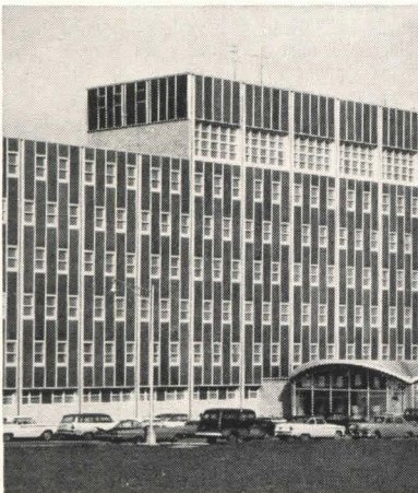
Western Pennsylvania State School & Hospital; Cannonsburg, Pa. Celli-Flynn, McKeesport, Pa.; Archt. & Engs. John McShain, Inc., Baltimore, Md.; Contr.
