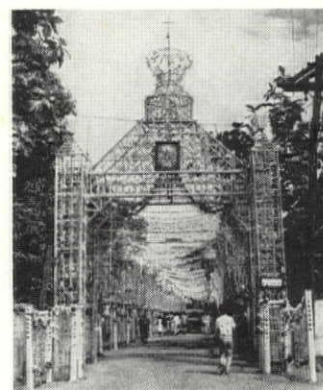
A fiesta arch (constructed of bamboo). Courtesy: The Manila Times
