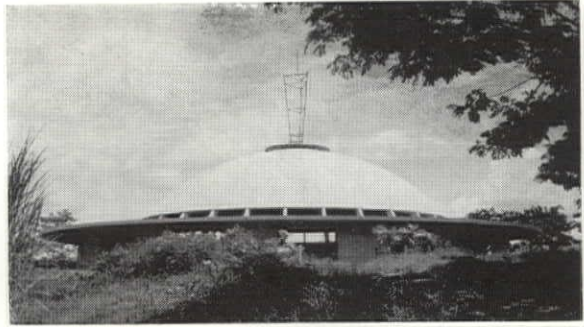
Chapel of the Holy Sacrifice at the University of the Philippines, Leandro V. Locsin, architect. The first 3" concrete shell dome in the Philippines, the church seats one thousand
