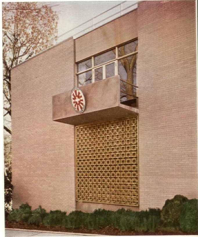
Embassy of Switzerland, Washington, D. C. (above and below). Bronze metals in sheet, rectangular tube, and extrusions were used by the fabricator to execute the architect's designs for spandrels, mullions, fascias, and columns. The grille (below), seemingly of solid bars, is actually fabricated from standard size, rectangular red brass tube. ARCHITECT: William Lescaze, New York. FABRICATOR: A. F. Jorss Iron Works, Arlington, Virginia.
