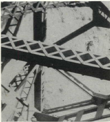
I couldn't help but be completely captured by the beauty of the falls. Even though they're criss-crossed with bridges, there is still something thrilling in this play of patterns—light and shadows of steel against the force of the water. LEWIS CRUTCHER
