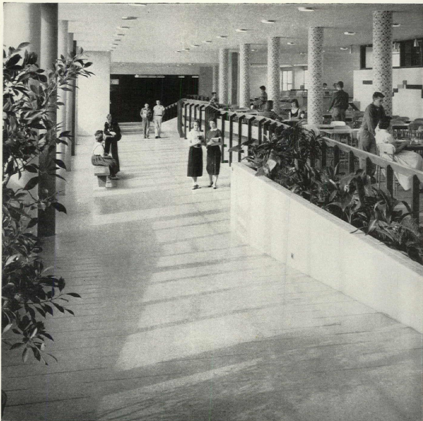
COMMONS CAFETERIA, COMO PARK JR. HIGH SCHOOL, MINNEAPOLIS, MINN. • PHOTO: WARREN REYNOLDS, INFINITY, INC., MINNEAPOLIS
