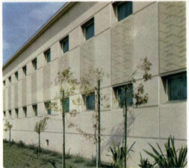
Architect: Arthur Goodman. Tile Contractor: Rigney Tile Co. Plate No. 550
