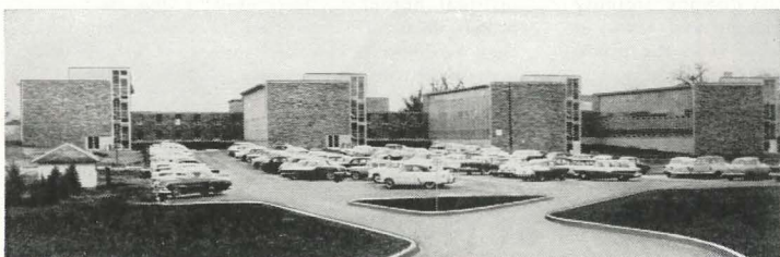
12,200 square feet of Porcelo Panels were used in the construction of the New Engineering Buildings at Colorado A. & M. College.
