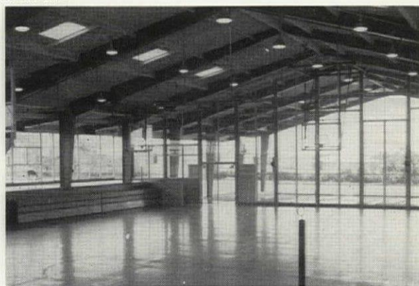
TYLER TEXAS JHS — GYM LOW END — NOTE SEATING
