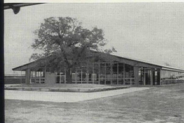
TYLER TEXAS JHS — GYM CAUDILL ROWLETT SCOTT ASSOCIATES, AIA
