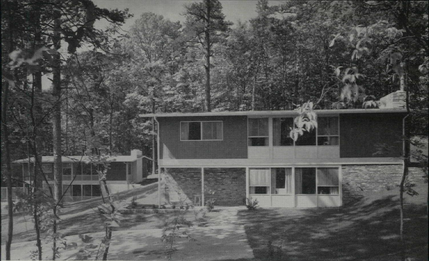
DEVELOPMENT HOUSES AT LAKE BARCROFT, VA. CONTEMPORARY HOUSES, INC., BUILDERS— KEYES, SMITH, SATTERLEE & LETHBRIDGE, ARCHITECTS
