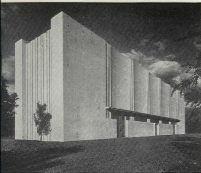
pumping station, Spokane, Wash.
