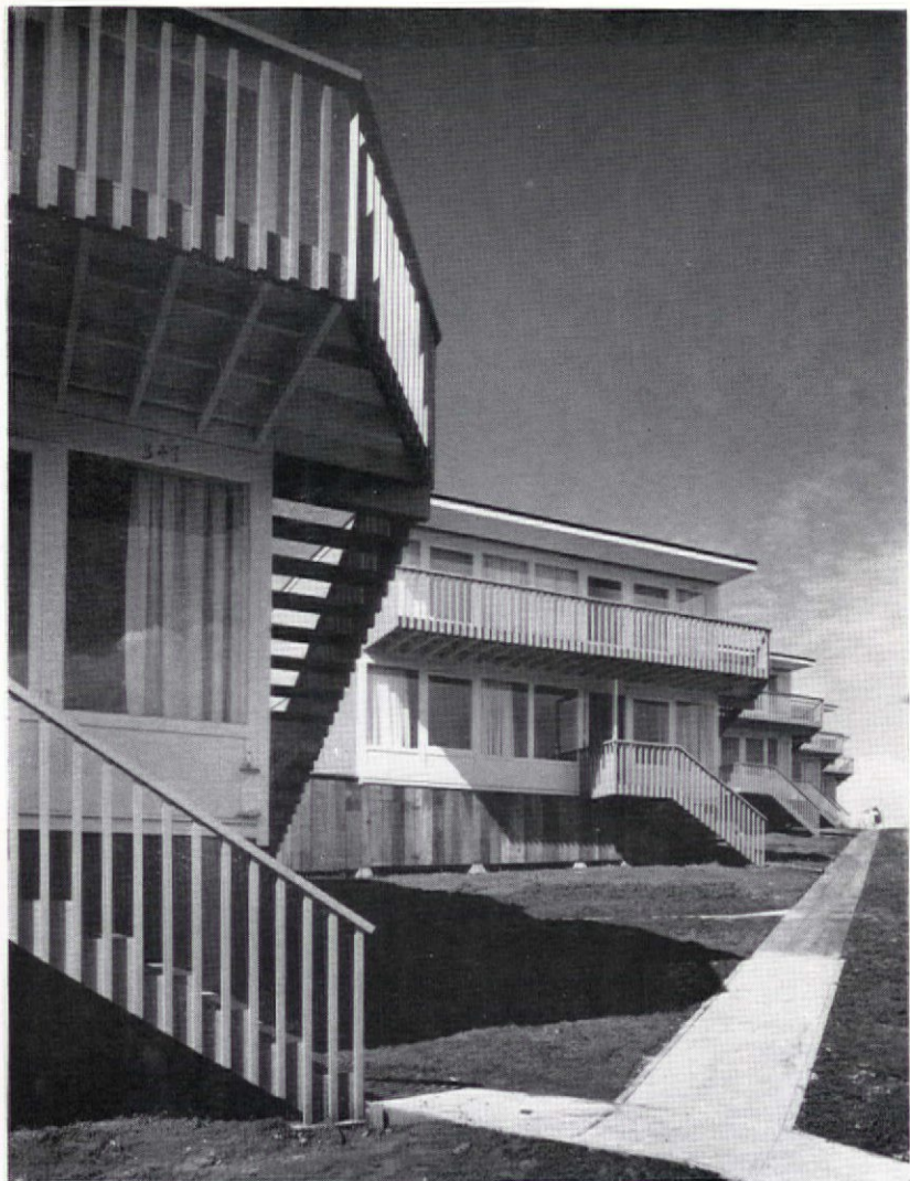
EXPERIMENTAL WAR HOUSING, COMPLETED 1942, VALLEJO, CALIF. WURSTER, BERNARDI & EMMONS, ARCHITECTS
