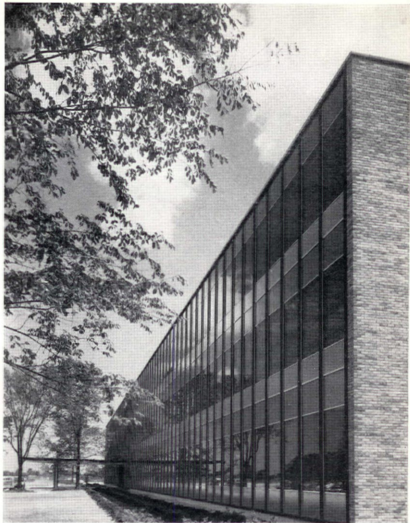
NORTH FAÇADE, GENERAL MOTORS TECHNICAL CENTER, WARREN, MICH.
