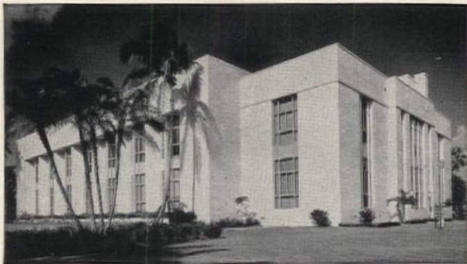
Miami Public Library —WHITE CHEROKEE VENEER MARBLE Architect —STEWART & SKINNER, MIAMI General Contractor —FRED HOWLAND, INC., MIAMI Marble Contractor —INTERSTATE MARBLE & TILE CO., MIAMI
