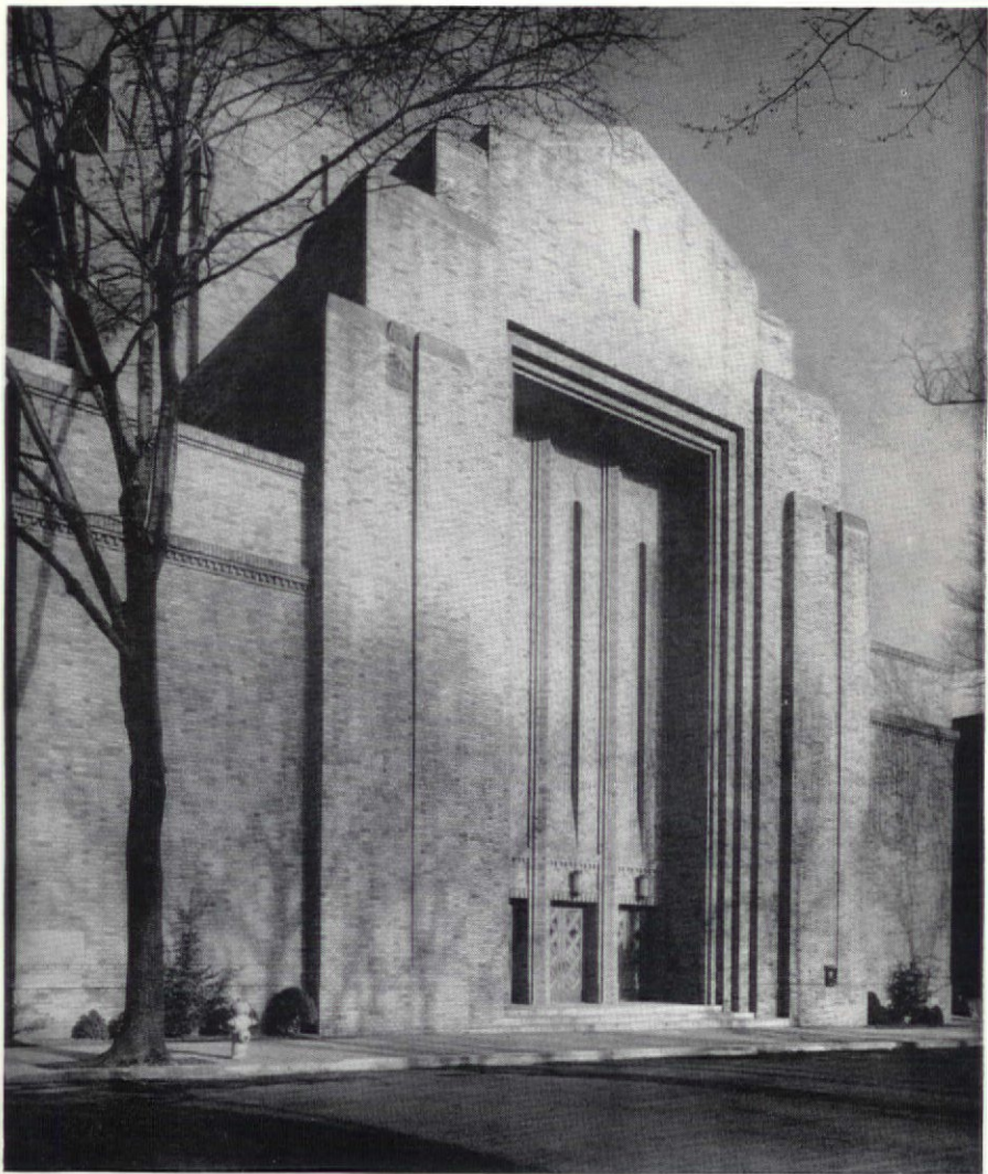
SIXTH CHURCH OF CHRIST, SCIENTIST, PORTLAND, ORE. ARCHITECTS: MORRIS H. WHITEHOUSE & ASSOCIATES— GLENN STANTON AND WALTER E. CHURCH
