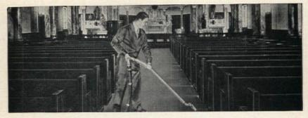
The vacuum producer and dirt container are located in the basement. Piping connects to convenient inlets all over the building.
