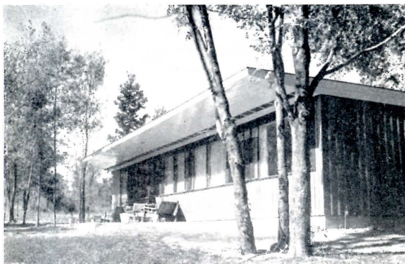
A RECENT HOUSE IN SHREVEPORT, LA. WILLIAM B. WIENER, ARCHITECT
