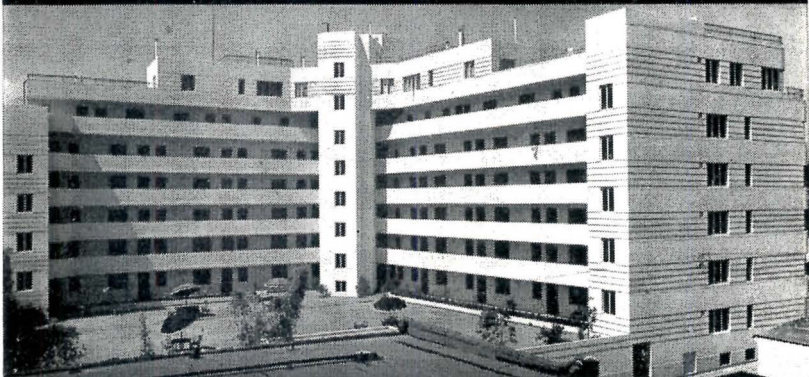
Shangri-La Apartments, Santa Monica, Calif., an example of the beauty and durability of architectural concrete construction. Wm. E. Foster, of Beverly Hills, architect; H. C. Whittlesey, structural engineer.
