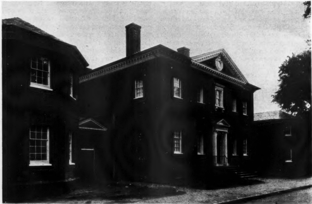
HAMMOND-HARWOOD HOUSE, ANNAPOLIS, MD.
