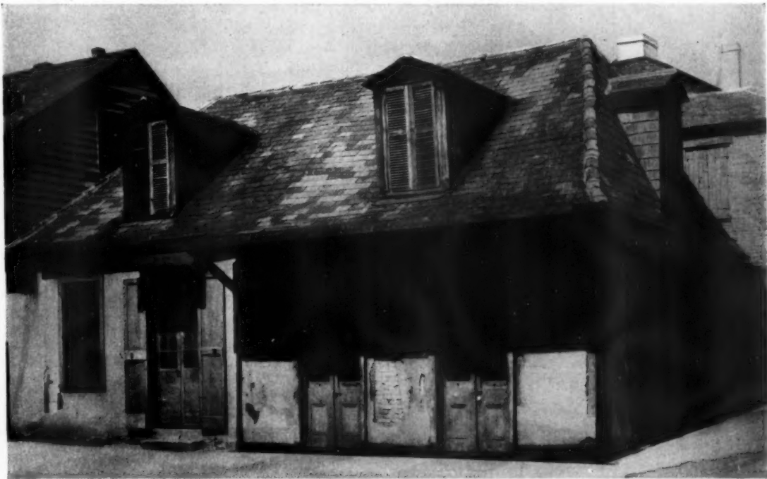
CORNER OF BOURBON AND ST. PHILIP STREETS "BRIQUETTES ENTRE POTEAUX" CONSTRUCTION
