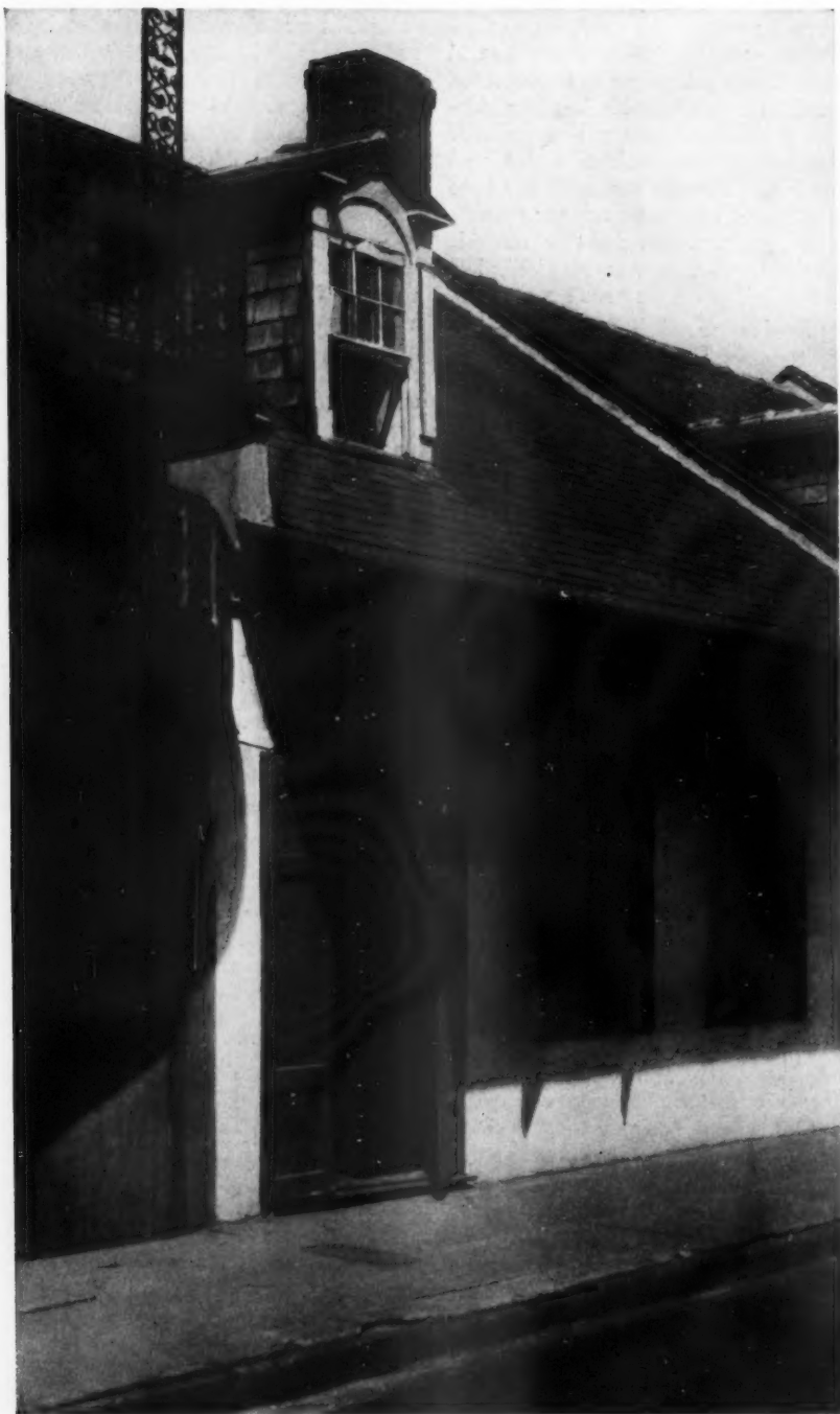
ON DAUPHINE STREET, NEW ORLEANS NOTE CORNICES. LIGHT WOODEN OVERHANGS SUPPORTED ON WROUGHT IRON BARS GIVE PROTECTION FROM SUN AND RAIN
