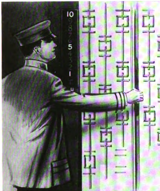
Illustrating a three-car installation in a ten-story building. Note Car No. 1 first floor, Car No. 2 fifth floor, Car No. 3 tenth floor.
