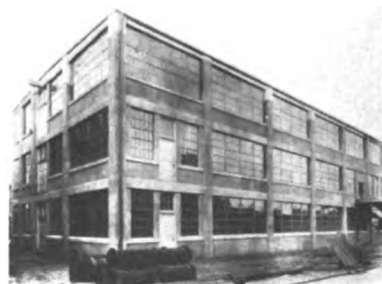
The plain factory building of reinforced concrete
