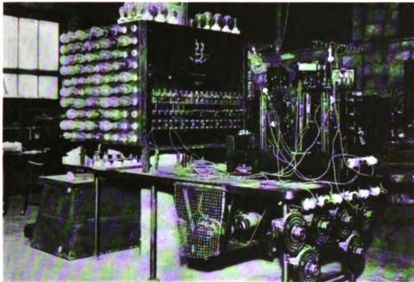
Switch and Socket Testing Machine
