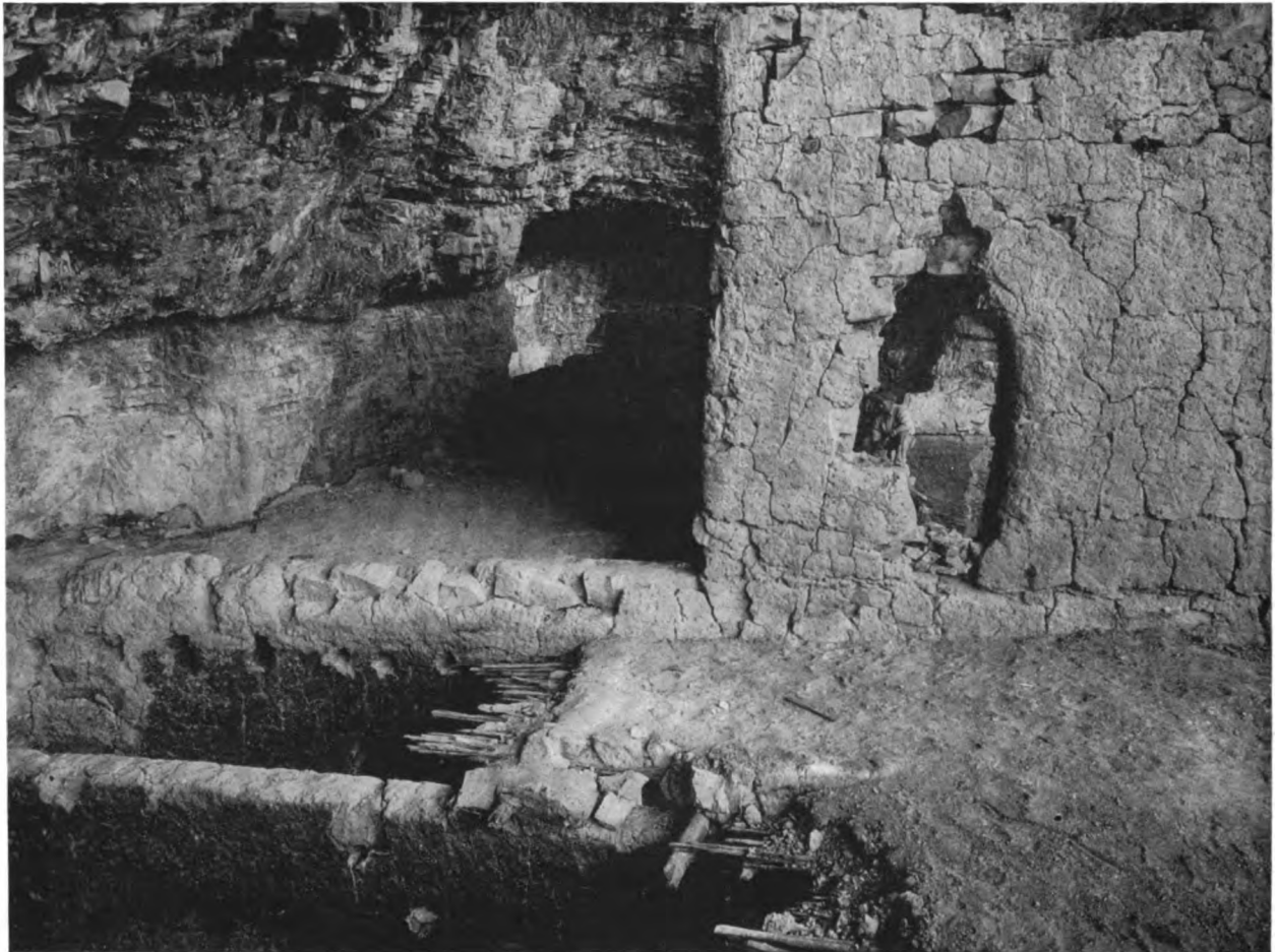
CLOSE VIEW OF A RUIN NEAR ROOSEVELT DAM, ARIZONA. The walls are of stone laid up in adobe mortar; some were plastered. The floor construction is of small, straight wands laid on cross-beams. Above these is placed the floor of stone and adobe. A man in the rear chamber may be seen through the hole in the wall.
