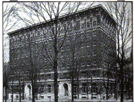
Y. M. C. A. Building, Grand Rapids, Mich. Architects: Robinson & Campau Gen. Contractors: Hauser, Owen, Ames Co. Rfg. Contractors: Geo. Van der Broek Co.
