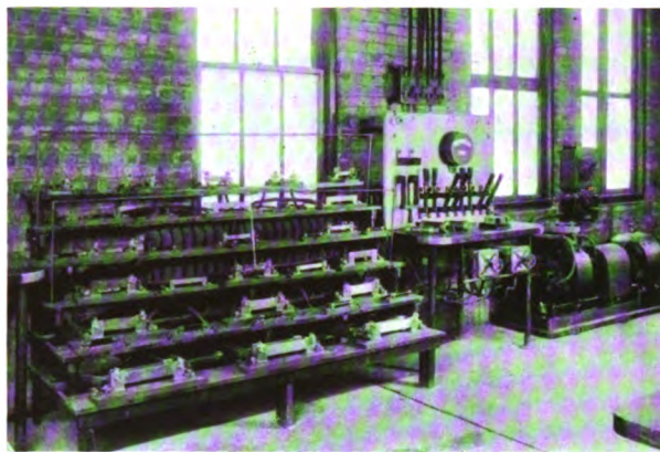
Circuits for Fuse Testing
