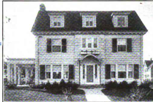
Architects, Shiner & Appel, New Haven, Conn. Owner, Wm. A. Thiel. Contractors, Lund & Lohne. 24-inch Shingles on side walls stained with "Dixie White" harmonize with moss-green roof and green blinds. A better effect than wide clapboards.
