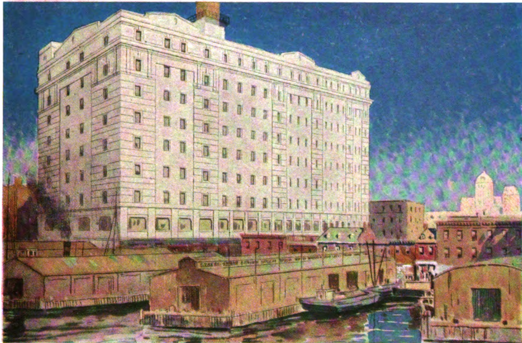
Reinforced Concrete Terminal Warehouse — Baltimore and Ohio Railroad, New York
