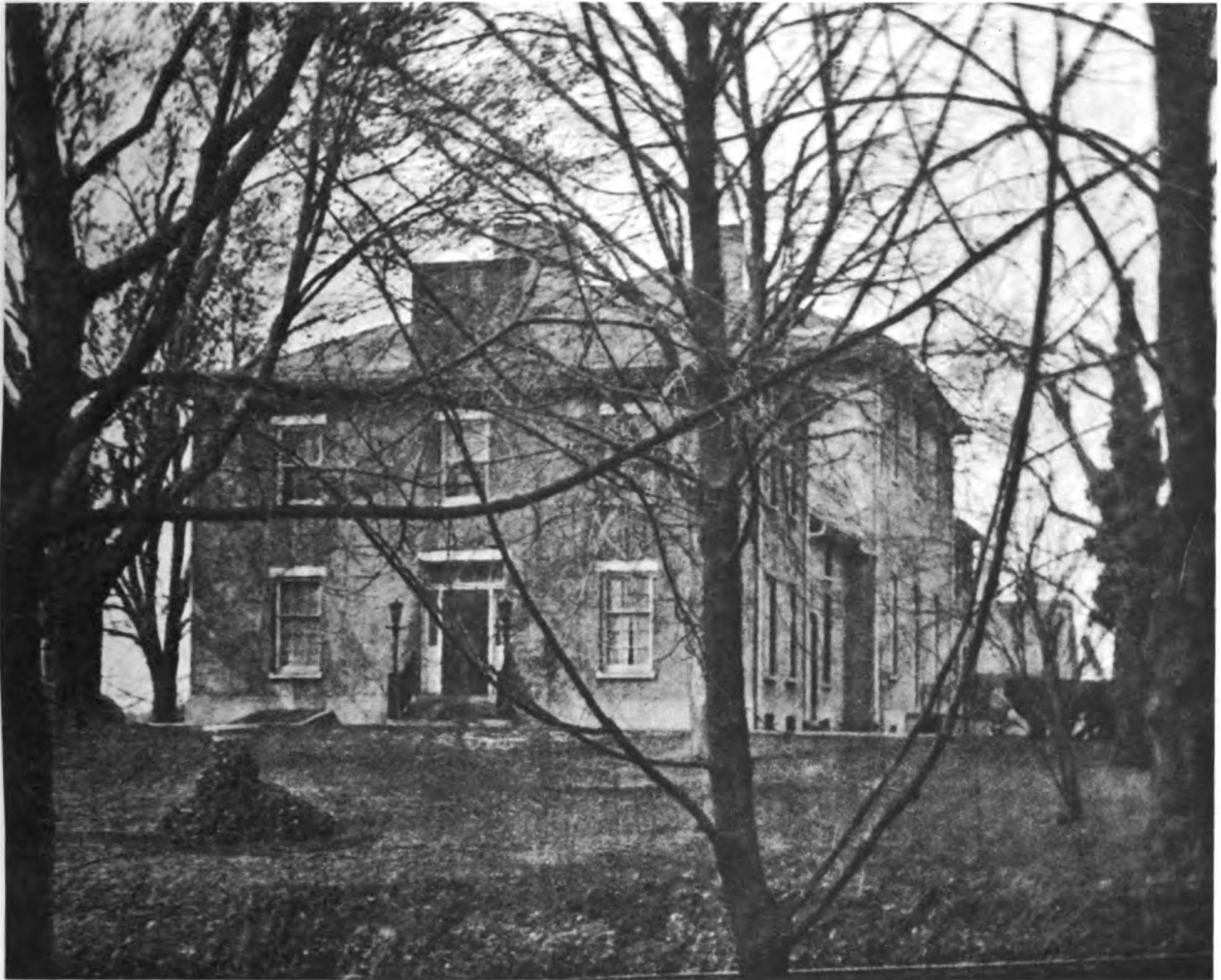
ON THE STUCCO WALLS OF TUDOR PLACE THE MORNING SUN WEAVES A FLEETING PATTERN OF BRANCH AND TWIG
