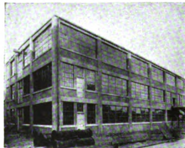
The plain factory building of reinforced concrete
