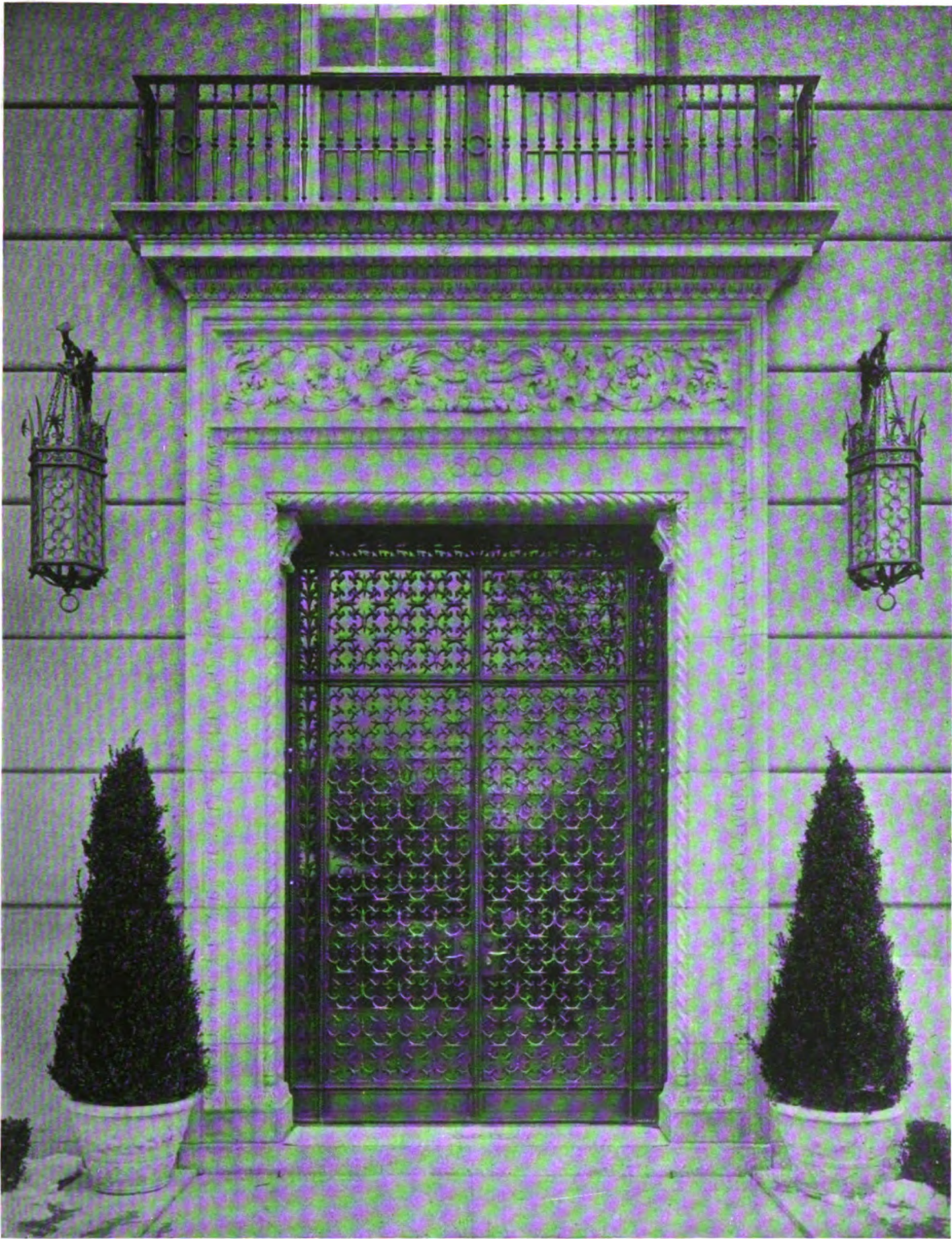
APARTMENT HOUSE, 63RD STREET AND FIFTH AVENUE, NEW YORK STARRETT & VAN VLECK, ARCHITECTS BRONZE ENTRANCE GRILLE, BALCONY RAIL VESTIBULE SCREEN, REGISTER FACES AND ELEVATOR DOORS EXECUTED BY
