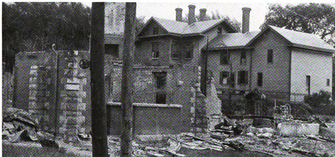
Shingle roofs spread the recent conflagration in Atlanta—Enough said!
