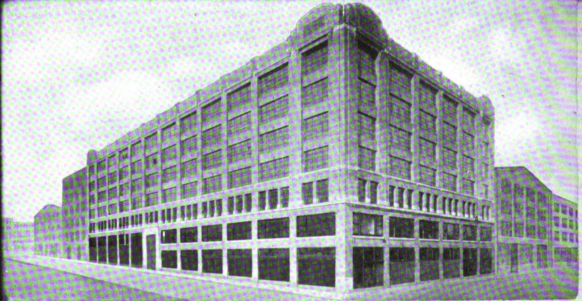
Kees &amp; Colburn Architects Foot-Schulze Building St Paul Minn Geo G Grant Construction Co Contractors
