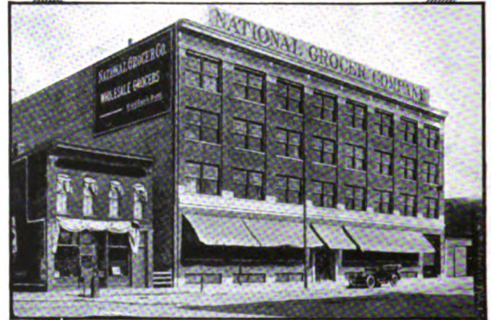
Caulfield Building, Grand Rapids, Mich. Architects: Wernette, Bradfield & Mead General Contractors: Horner & Kelly Roofing Contractors: Eikenhout & Sons Co.
