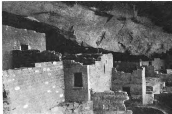
The skill with which the hewn stones were laid in Cliff Palace is well illustrated here. Note the projecting window-sill and the preserved condition of the wall.
