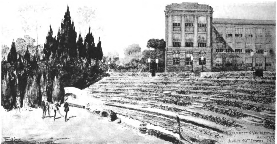
MONTCLAIR, N. J. A GARDEN THEATRE.—THE AUDITORIUM WITH BENCHES REMOVED
