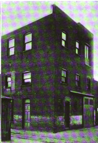
Department of Agriculture Bureau of Chemistry, Storage Rear of 215 Twelfth Street, S. W. Assessed value, $3,483.00; real value, $5,225.00; *annual rental, $600.00; †net return to owner, 10.75%.
