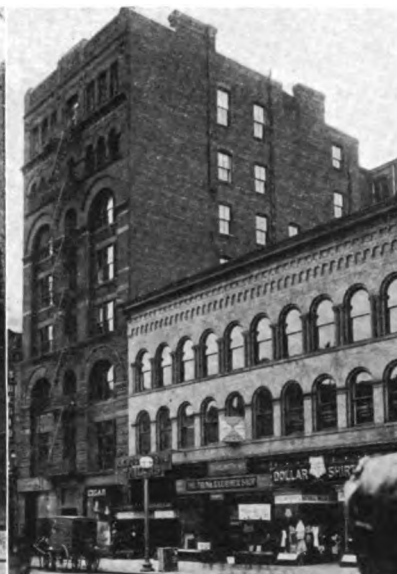
Department of Agriculture Forest Service Atlantic Building, 929 F Street, N. W. Assessed value, $138,670.00; real value, $209,000.00; annual rental $18,000.00. Other rentals in the building are $3,120.00 per annum. An apparently fair rental, but the building is a dangerous fire risk.
