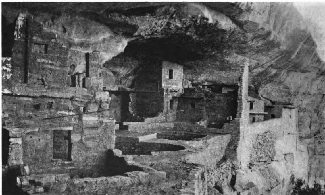
Balcony House shows the only example of balcony construction. The balcony is seen to the right of the picture. The parapet wall in front of the balcony overhangs a depth of several hundred feet. The circular chambers in the foreground are kivas, over which the floor of the terrace once existed. Note the stone lintel of the window.
